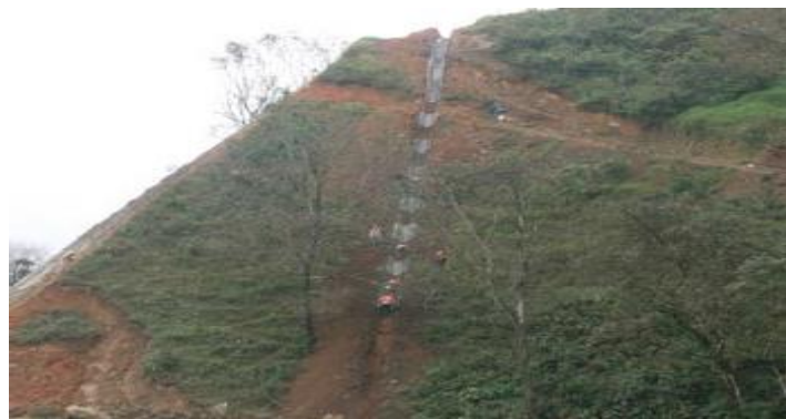
Figure 33 and 34: Drainage systems were implemented to control runoff and maintain the hydrological system. Source: CONNET. El Proyecto Mantendra La Conexion Hidrologica de La Zona . Photo report, n.d.
