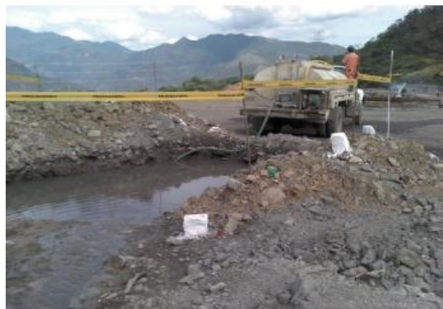
Figure 27 and 28: Water catchment areas were excavated to store runoff or surface waters for later use during construction. Source: CONNET. El proyecto mantendra la calidad del agua . Photo report, n.d.
