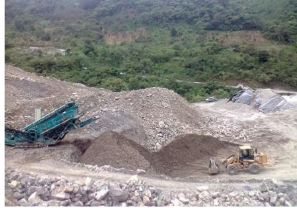
Figure 58 (left) and Figure 59 (right). A gravel crusher uses the extracted rock material to be reused in the project. Source: CONNET. Planta Trituradora . Photo report, n.d.
