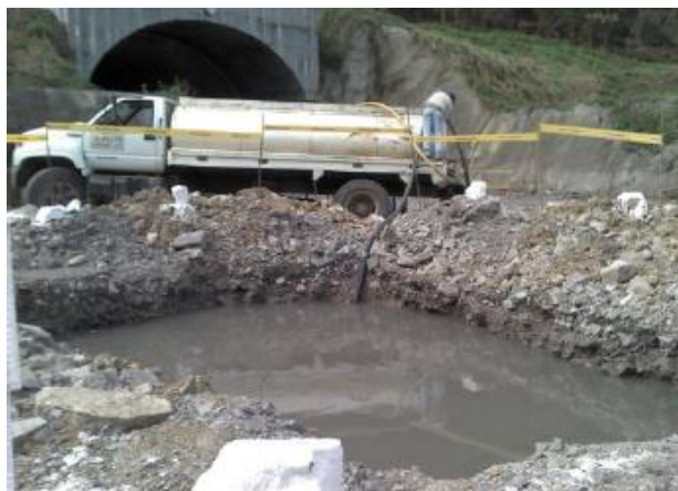
Figure 27 and 28: Water catchment areas were excavated to store runoff or surface waters for later use during construction. Source: CONNET. El proyecto mantendra la calidad del agua . Photo report, n.d.
