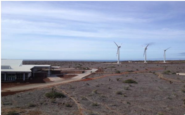
Figure 21: Wind turbine /Source: LEED Wind Turbines L-17.3_EA6
