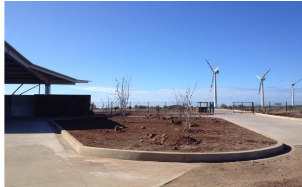
Figure 22: Wind turbine /Source: LEED Wind Turbines L-17.3_EA6
