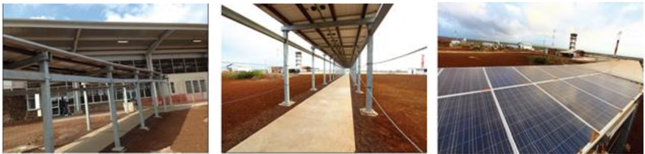
Figure 20: Use solar panels to shade some of the external paths/ Source: Energy and Atmosphere, page, L-13-3; credit SS- 7.1 , EA-2
