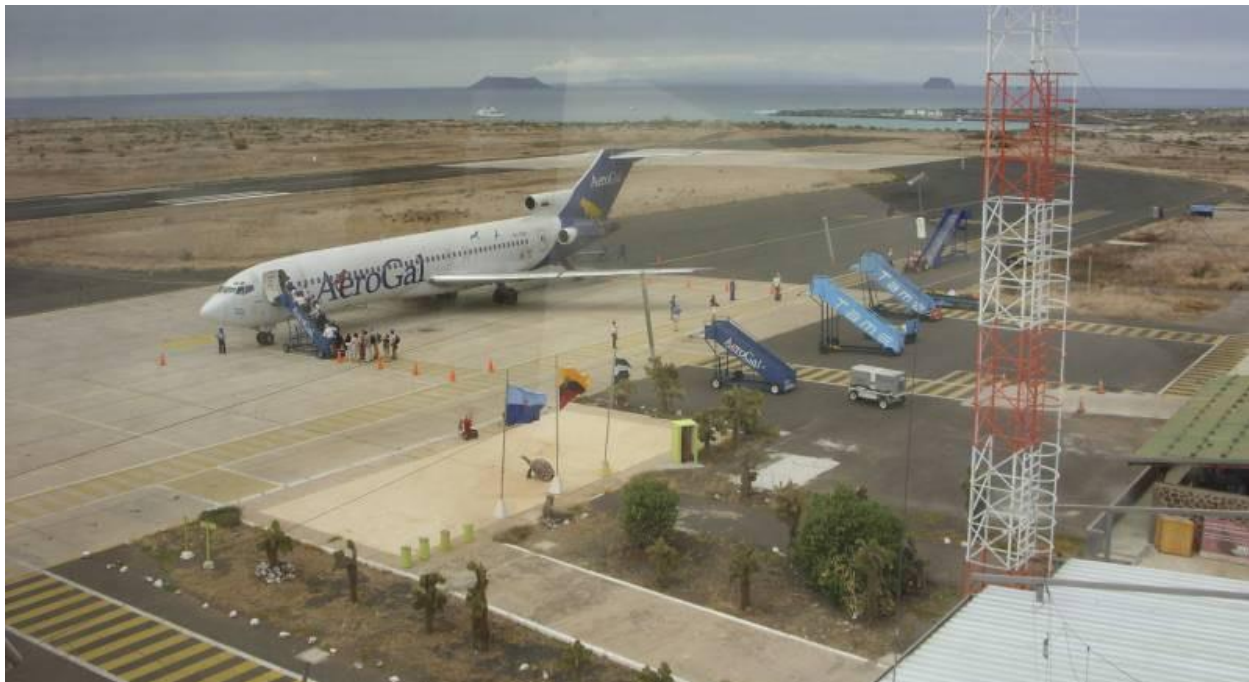
Figure 01: Ecological airport, platform view. \ Source: Environmental Impact Assessment, page 38, figure 3-4
