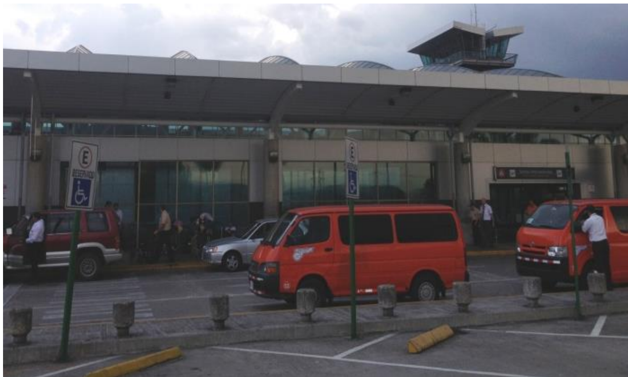
Figure 12: Main terminal entrance. Source: Picture taken during onsite visit, April 2013
