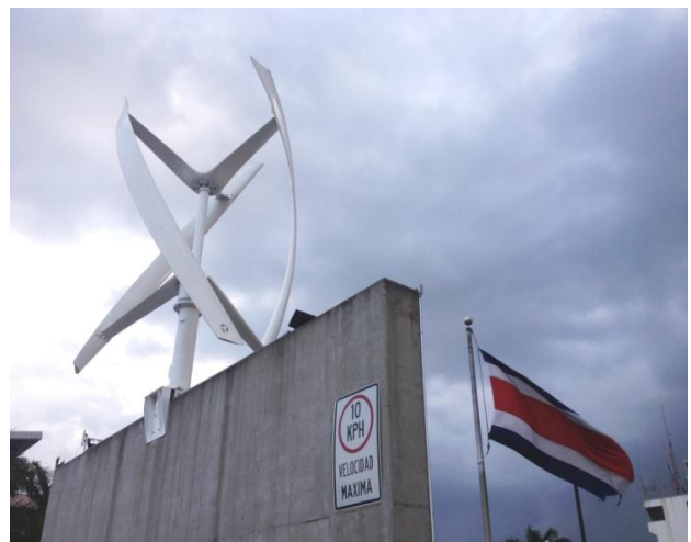
Figure 30: Windmill located in the parking
