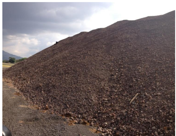
Figure 24: Re-use of excavated material. Source: Picture taken during onsite visit, April 2013
