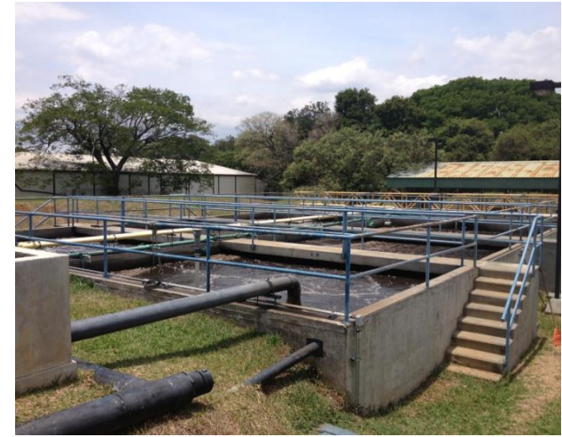
Figure 18: Water treatment plant.
