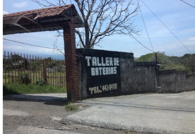
Figure 50: Industries surrounding the river. Source: Picture taken during onsite visit, April 2013
