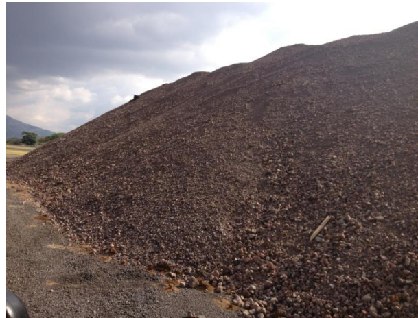
Figure 2: Re-use of excavated material
