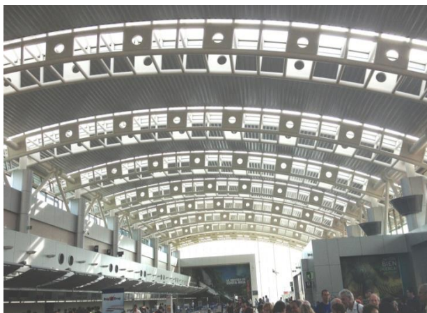
Figure 31: Natural lighting allows for electricity savings. Source: Picture taken during onsite visit, April 2013
