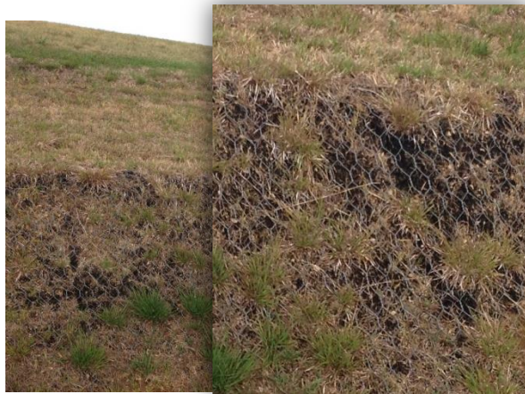
Figure 55: Measures to prevent landslides. Source: Picture taken during onsite visit, April 2013
