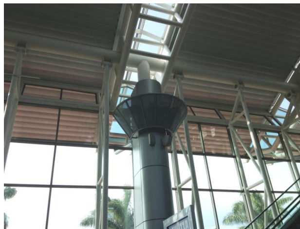
Figure 23: Illumination of the terminal.
