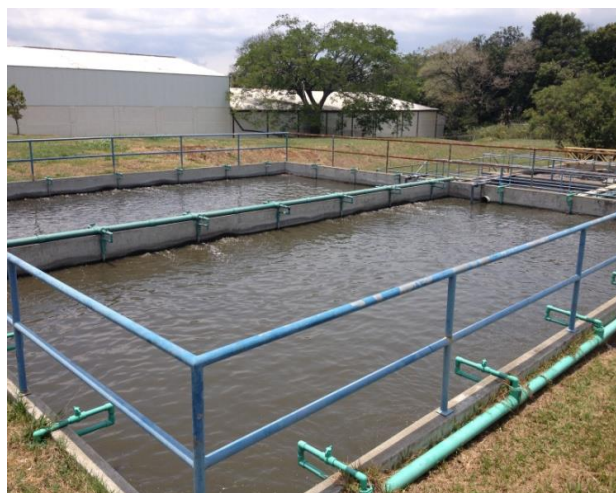
Figure 17: Water treatment plant.
