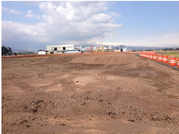
Figure 1: Re-use of excavated material
