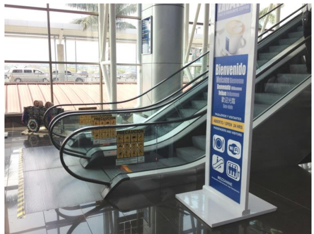
Figure 24: Stairs stop when there is no public
