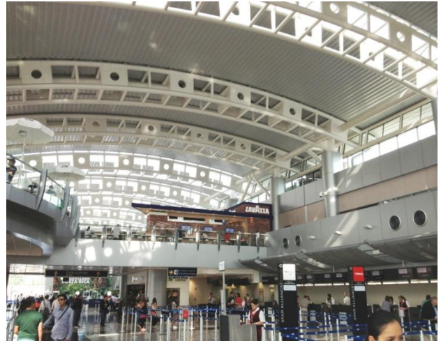
Figure 22: General view of the terminal.
