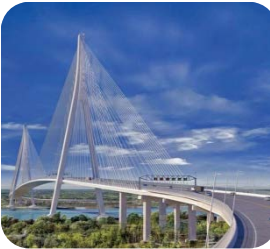
Gordie Howe International Bridge Detroit, MI
