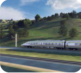
California High-Speed Rail Program (Phase I) Sacramento, CA
