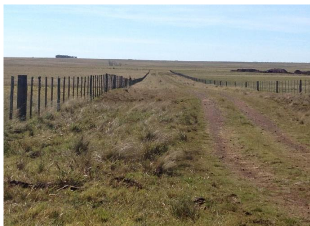
Figure 22: View of the state of paths before their improvement Source: Picture taken during the onsite visit May 2013
