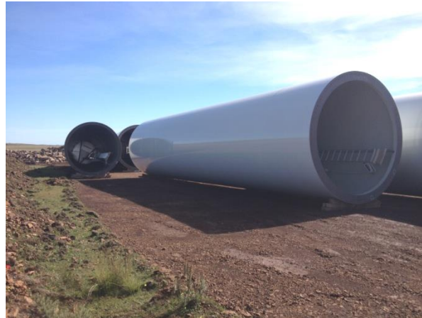
Figure 28': Stockpiling of the towers.
