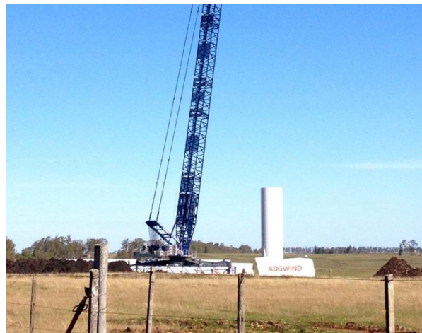
Figure 10': Wind turbine assembly
