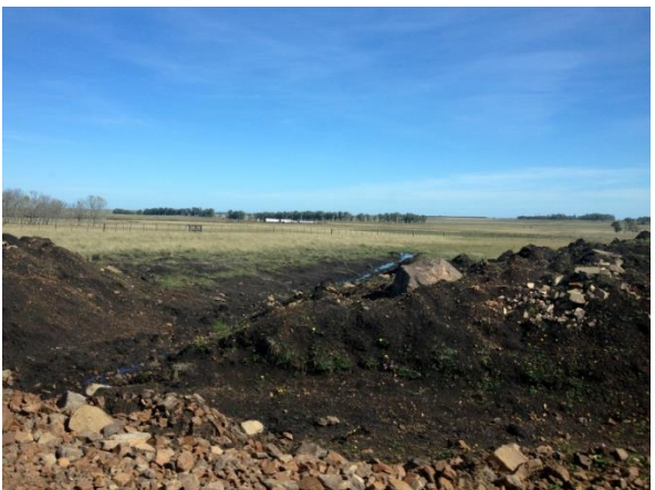
Figure 6': Excavated soil to improve the paths
