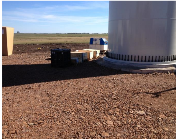
Figure 8': Filling and compacting of the excavated area
