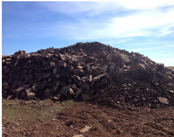
Figure 29: Reuse of excavated material. Source: Picture taken during the onsite visit May 2013
