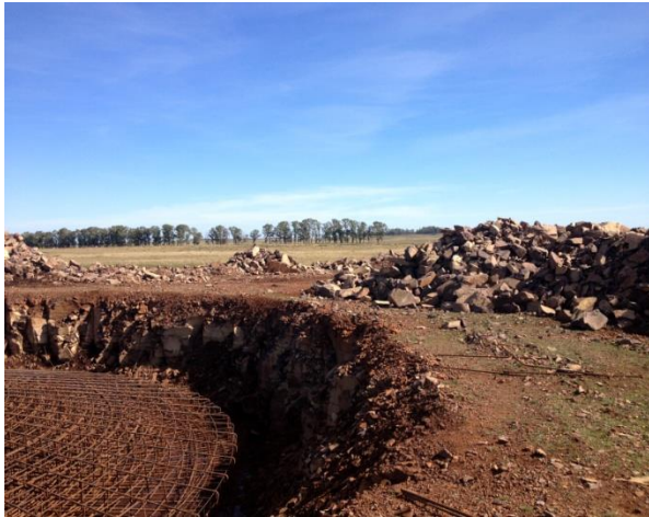
Figure 7': Foundation's excavation and stockpiling of soil for later reuse
