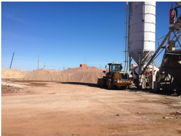
Figure 15': On site concrete plant
