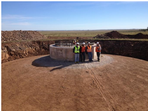
Figure 30': View of one of the foundations
