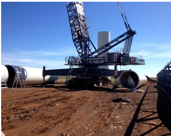
Figure 9': wind turbine assembly
