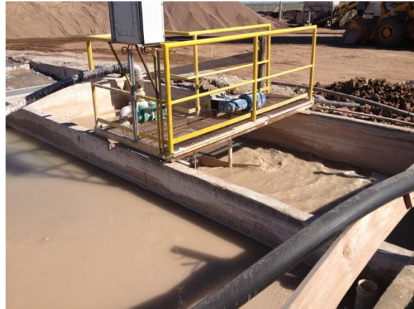
Figure 14': On site concrete plant
