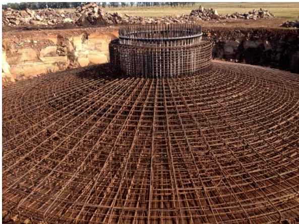
Figure 29': View of one of the foundations
