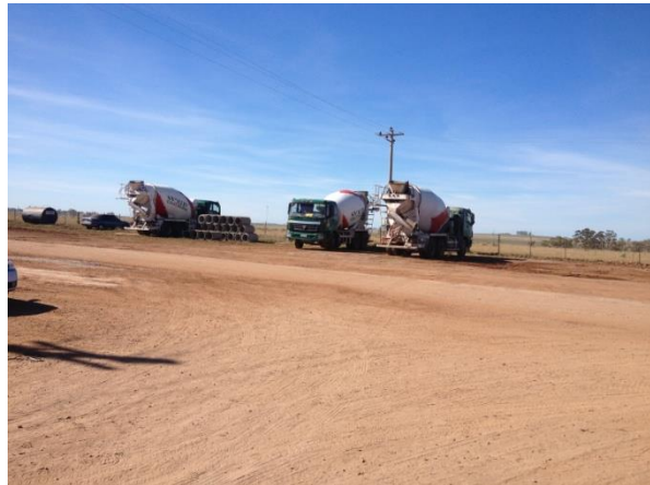
Figure 16': On site concrete plant
