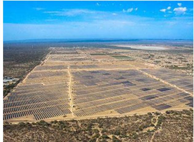
Figure 49 Aerial View of Photovoltaic Plant Source: Aura Solar, Línea de Tiempo, p. 10.
