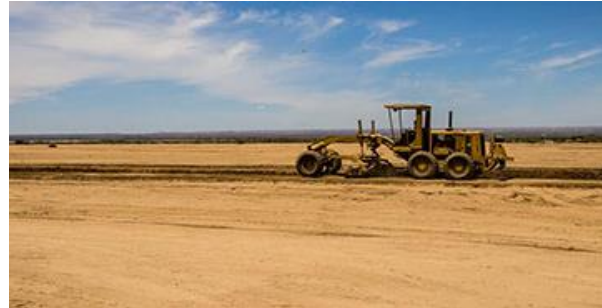
Figure 25: Leveling of terrain in project site
