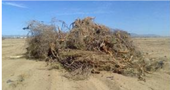
Figure 24: Recollection of herbs and shrubs for site leveling
