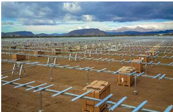
Figure 44: Photovoltaic Modules' Structure Installation Source: Aura Solar, Línea de Tiempo, p. 6.
