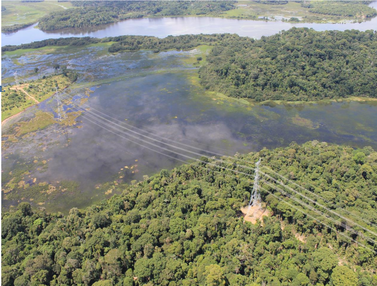
Figure 01: General view of the transmission line / Source: ISOLUX CORSÁN
