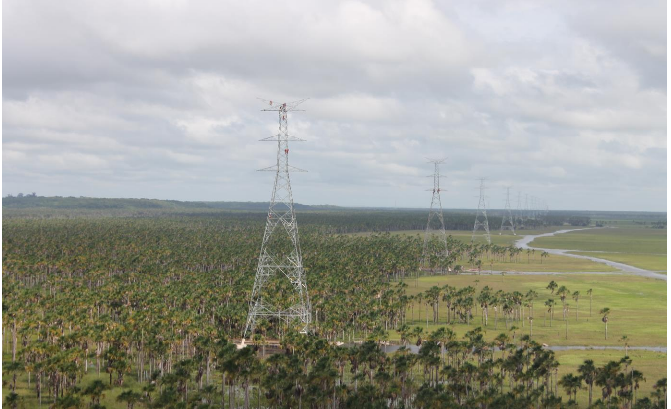
Figure 37: General view of the transmission line. /Source: Isolux Corsán
