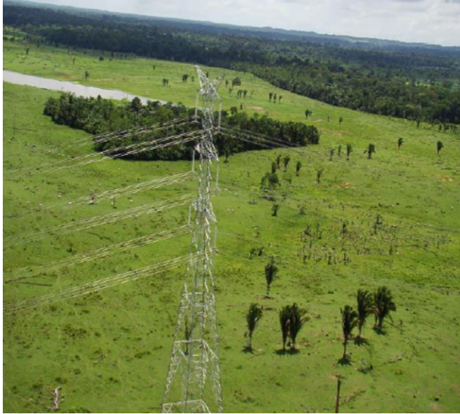
Figure 27: Whenever possible the HTL was deployed on areas previously affected by man-made activities. Source: Isolux Corsán
