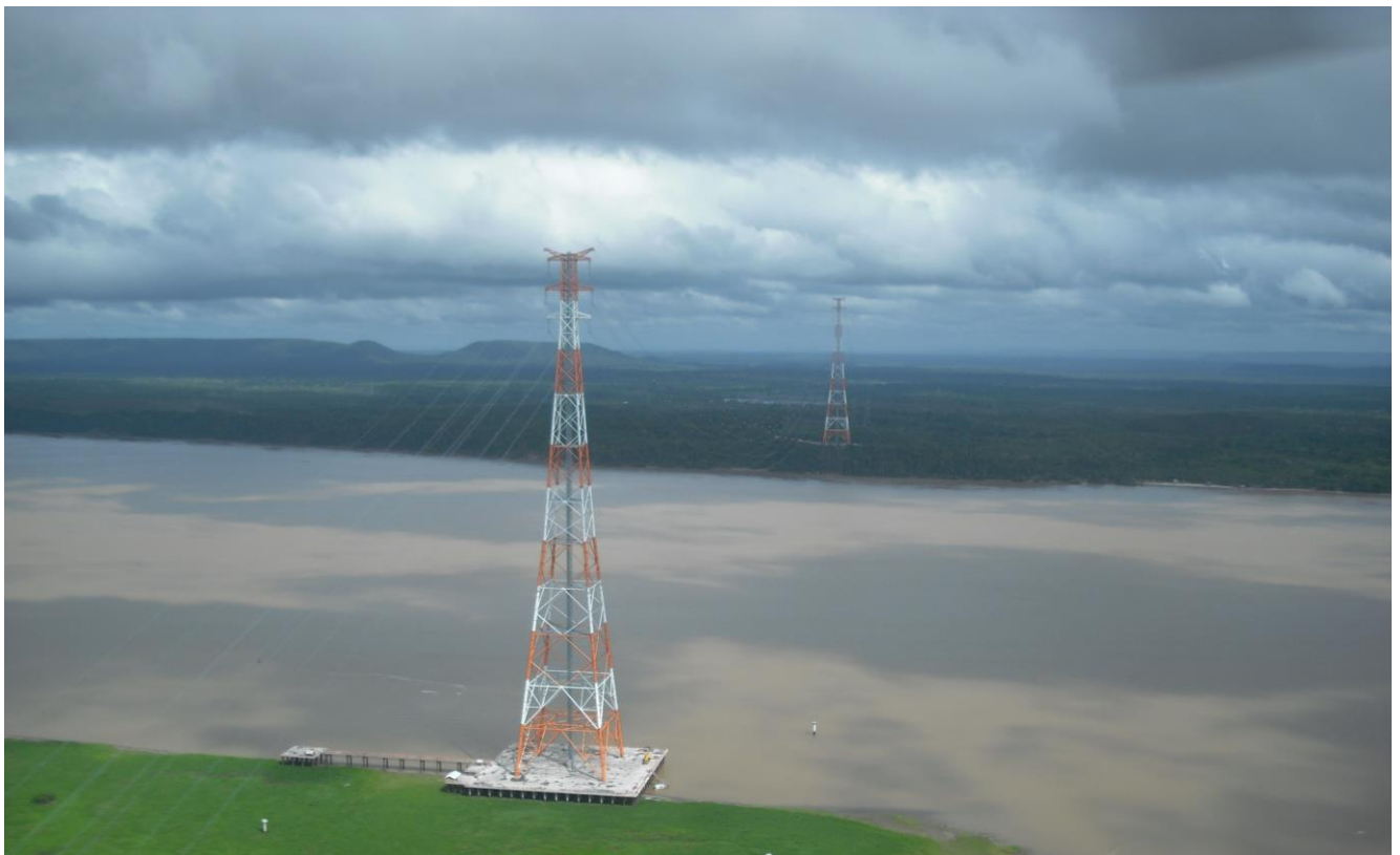
Figure 29: High Tension Towers at the Amazon River / Source: Isolux Corsán
