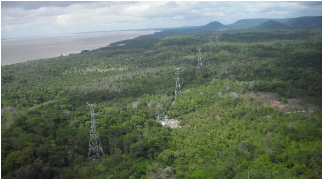
Figure 31: General view of the transmission line / Source: Isolux Corsán
