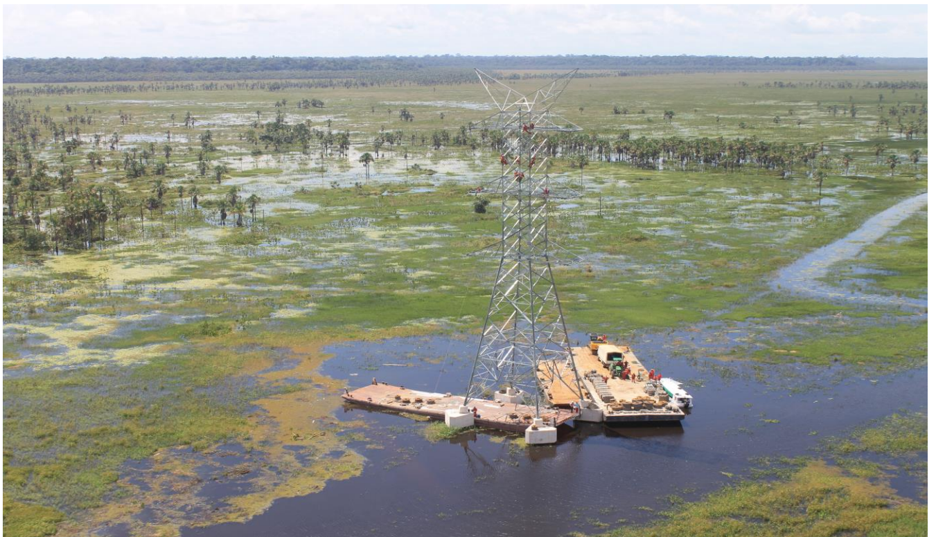
Figure 38: High Tension Towers during construction / Source: Isolux Corsán
