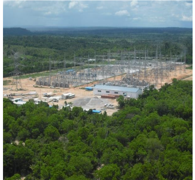
Figure 28: view of the site /Source: Isolux Corsán
