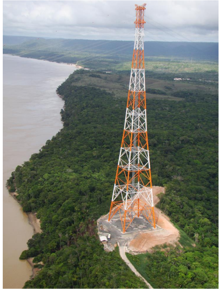
Figure 33: High Tension Towers at the Amazon River / Source: Isolux Corsán
