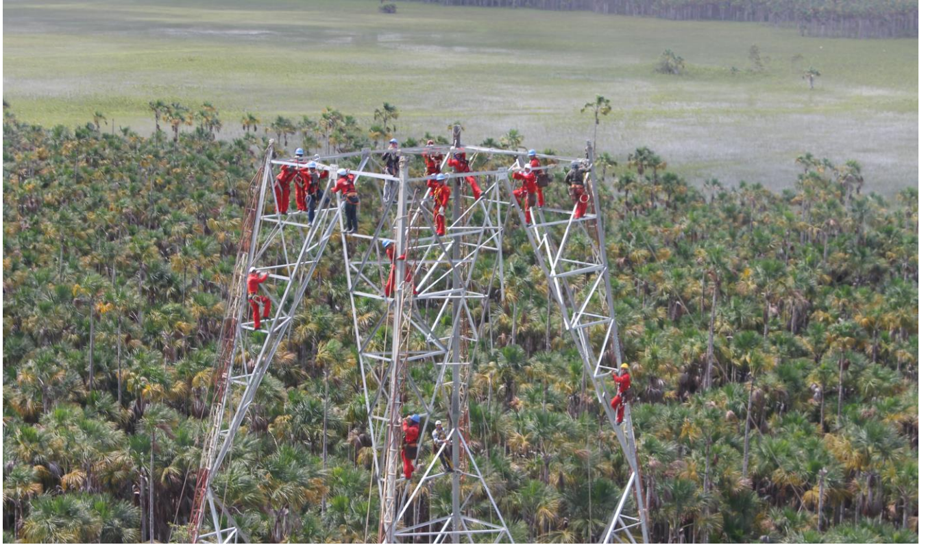
Figure 39: High Tension Towers during construction / Source: Isolux Corsán
