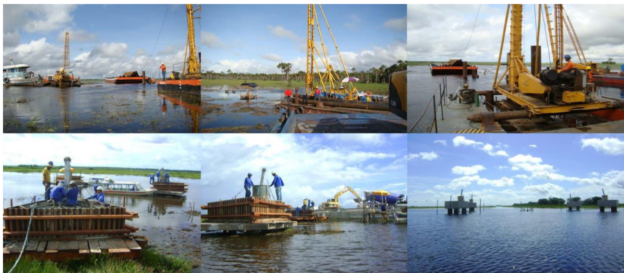
Figure 17: Deployment of Infrastructure in flooded areas./ Source: Isolux Corsán.
