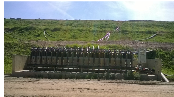
Figure 26: LFG collecting system. Sources: Image sent from CTR Rio project team
