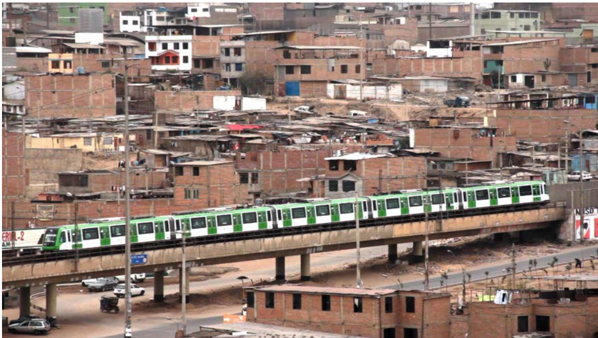
Figure 42: L1ML's Section 1 rail viaduct in Villa Maria del Triunfo district / Source: L1ML
