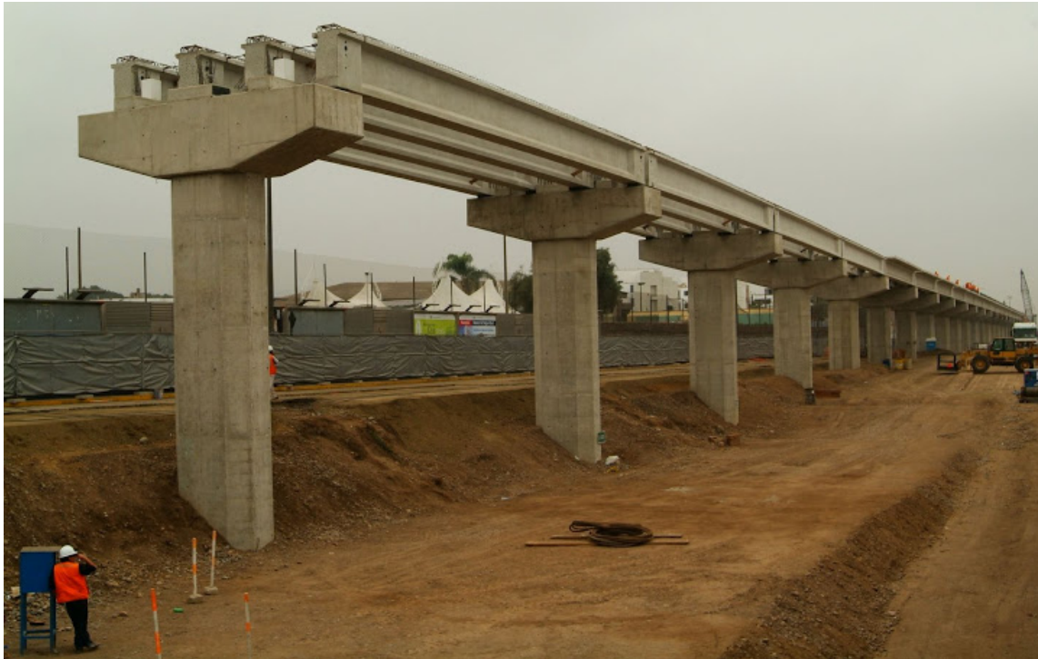
Figure 74: L1ML prefabricated superstructure
