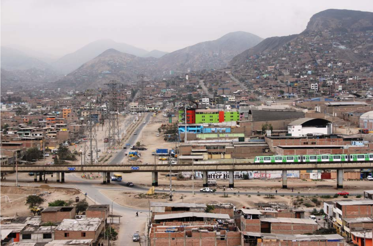
Figure 44: L1ML's Section 1 rail viaduct in Micaela Bastidas neighborhood association, Villa Maria del Triunfo district / Source: L1ML
