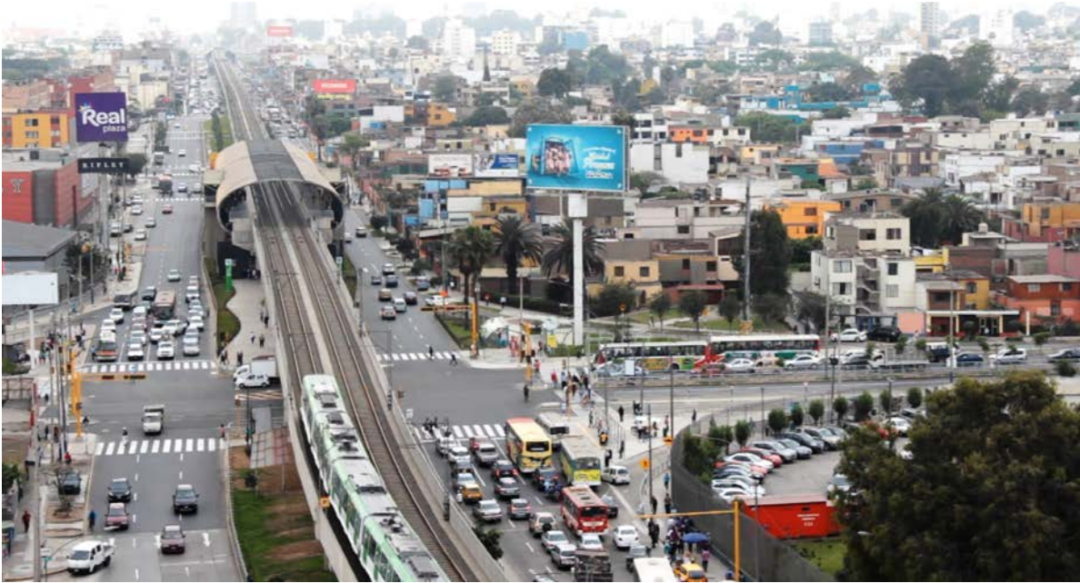
Figure 41: L1ML's Section 1 station and rail viaduct in Villa Maria del Triunfo district / Source: L1ML
