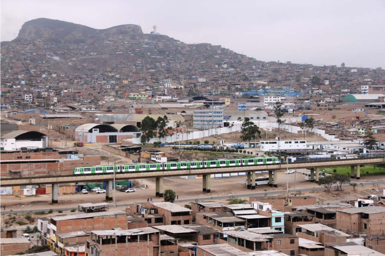
Figure 43: L1ML's Section 1 rail viaduct in Micaela Bastidas neighborhood association, Villa Maria del Triunfo district / Source: L1ML
