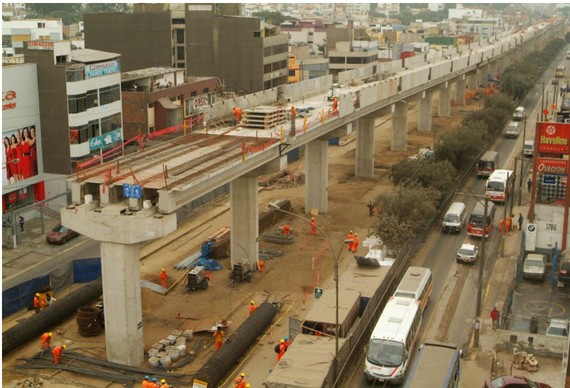
Figure 75: L1ML viaduct in central avenues berm
