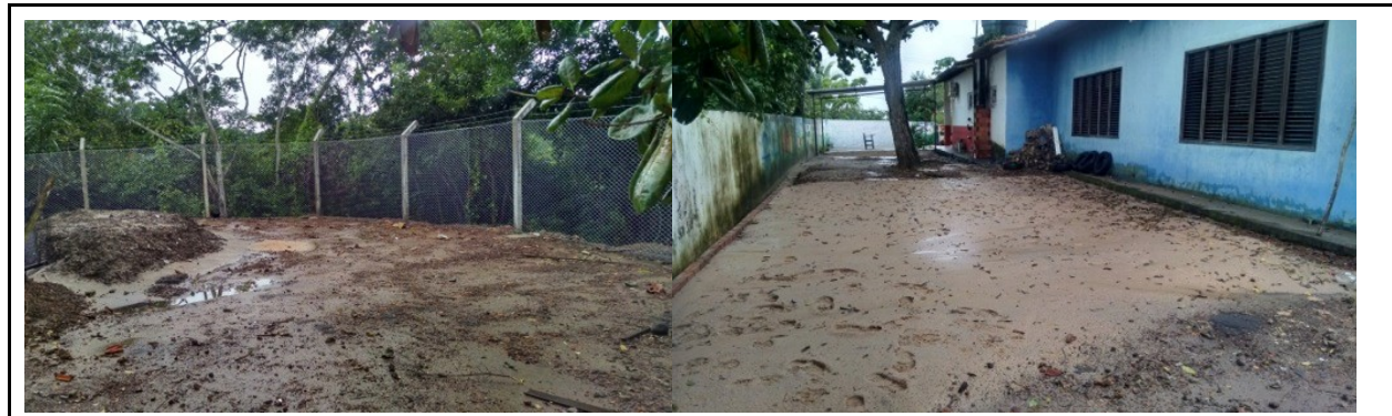
Figure 14: Josefina Serrão School patio area destined for the plantation of an orchard Sources: TEGRAM, Relatório de Andamento 4 (São Luís, MA: 2015).
