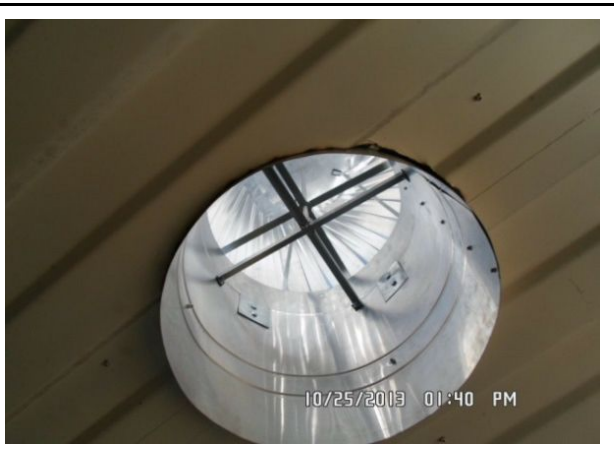
Figure 17: Wind Extractor Energy Producer Sources: Pert, "Informe Seguimiento a la Gestión en HSEQ". (Internal Document Puerto Bahía, Unknown Location and Date). 23.
