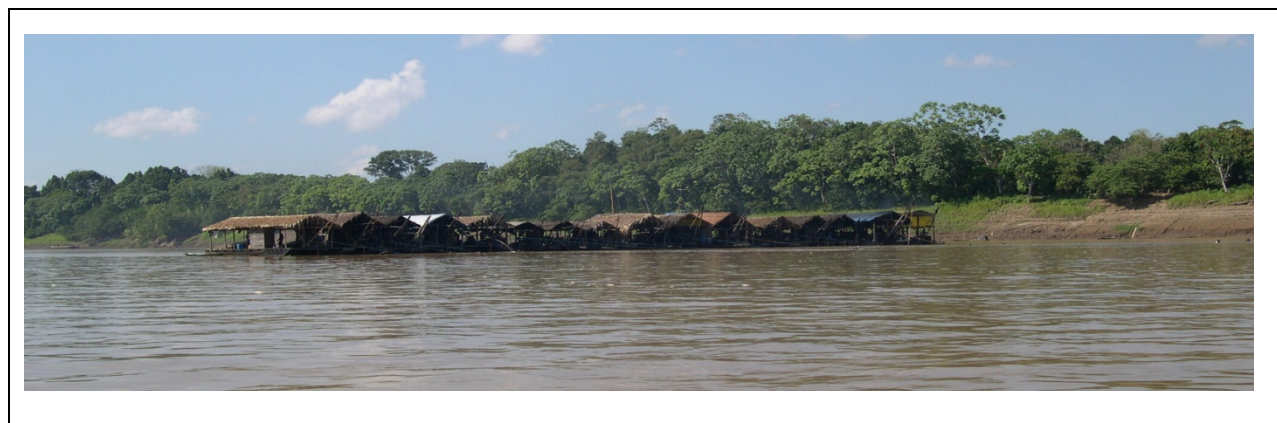
Figure 08: Typical structures on the water Sources: Santo Antonio Energia and EQAO, Santo Antonio Hydropower Project (2014).
