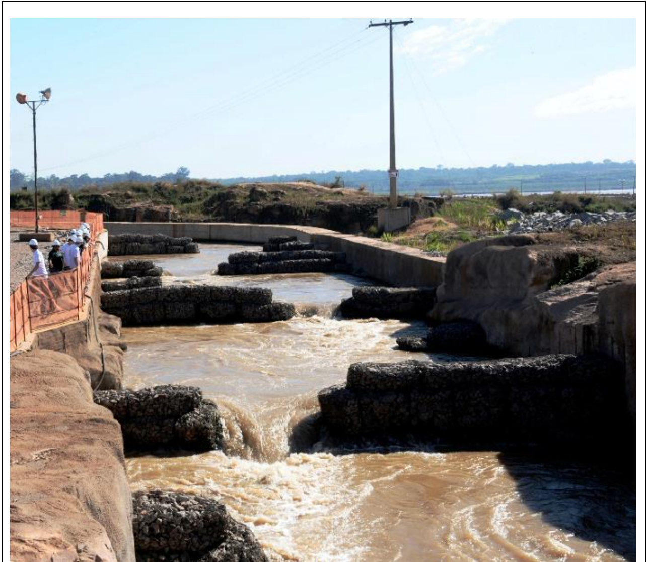
Figure 05: Fish Transposition System Sources: Santo Antonio Energia and EQAO, Santo Antonio Hydropower Project (2014).
