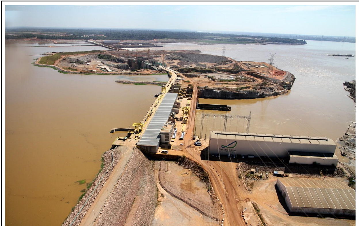
Figure 01: General picture of Santo Antonio hydroelectric plant. Sources: Santo Antônio Energia
