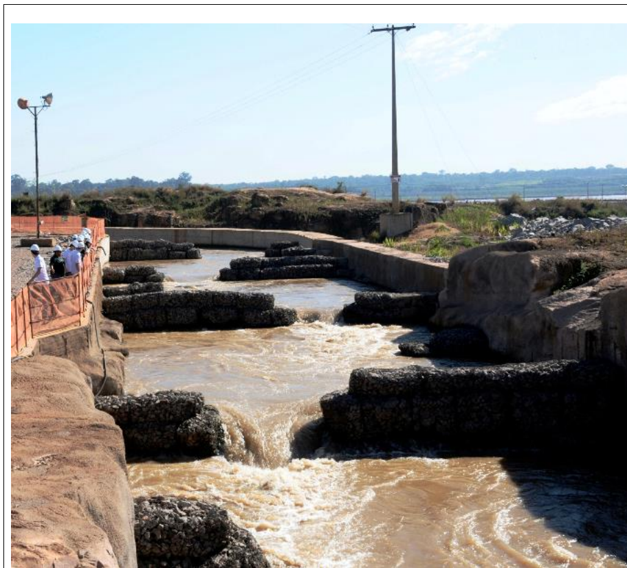
Figure 05: Fish Transposition System Sources: San Antonio Energia and EQAO, San Antonio Hydropower Project (2014).
