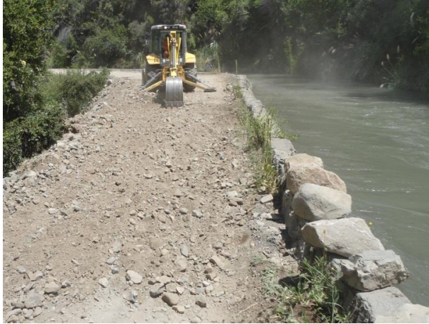
Figure 14: improvement of canal edge. Picture provided by Besalco S.A.
