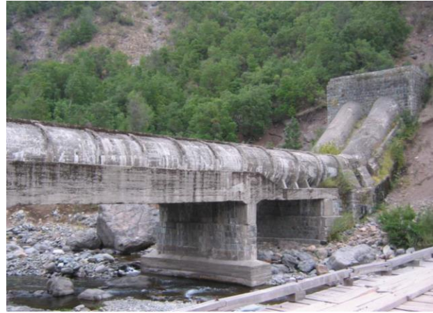
Figure 52: "El Melado Canal", siphon "El Toro", 1.2 km route.
