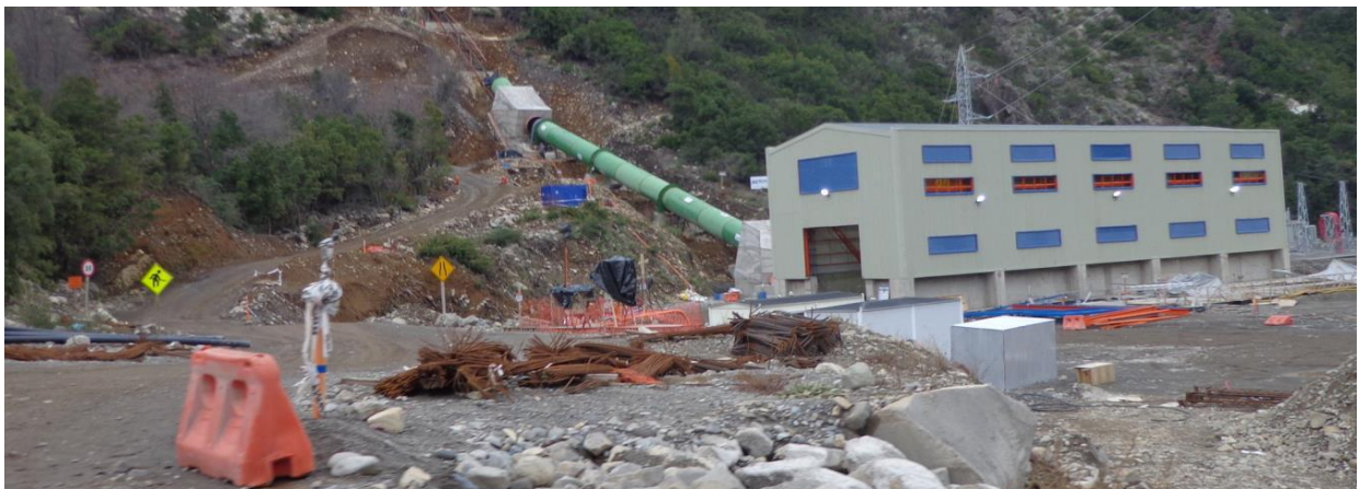
Figure 53: signage in the works area. Picture provided by Besalco S.A.
