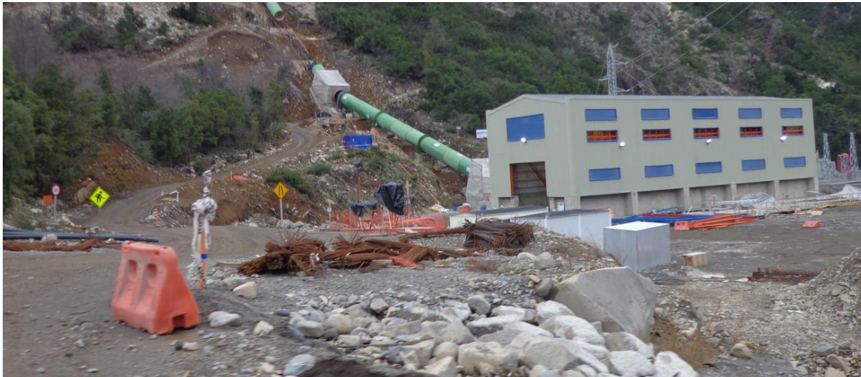
Figure 16: signage in the works area. Picture provided by Besalco S.A.
