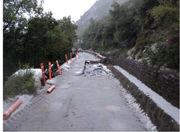
Figure 15: improvement of canal edge. Picture provided by Besalco S.A.
