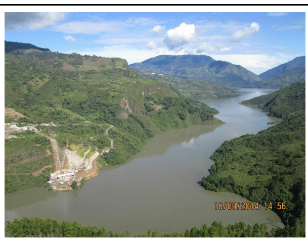
Figure 12: Esmeralda reservoir pictured after water level rise. Source: Fotos AES Chivor
