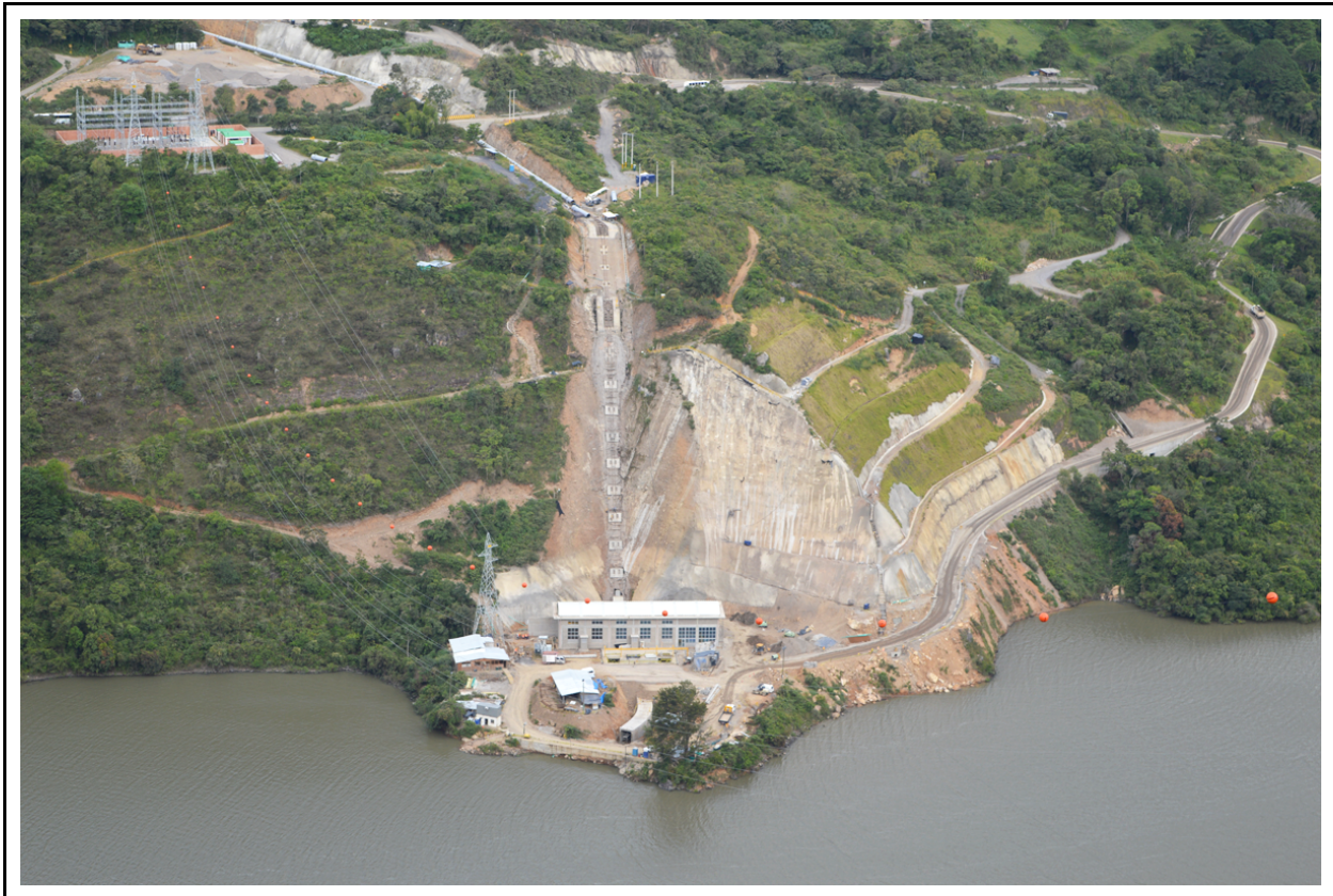
Figure 01: Machine house under construction Source: Fotos AES Chivor
