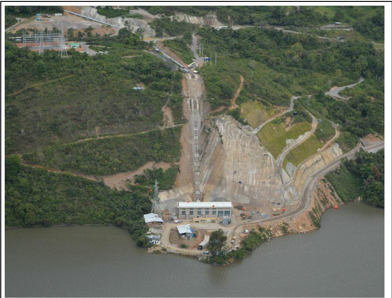
Figure 02: View from above machine house Source: Fotos AES Chivor
