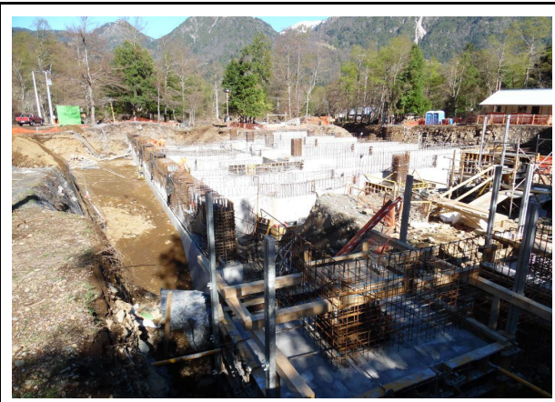
Figure 15: Construction process Sources: Pictures provided by LAP
