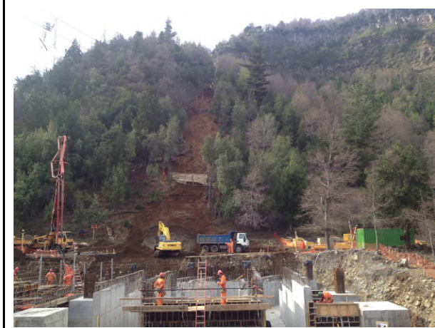
Figure 18: Construction process Sources: Pictures provided by LAP
