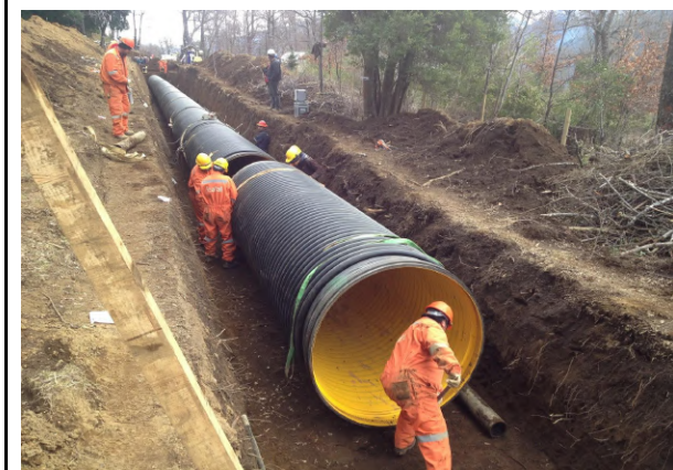
Figure 16: Construction process Sources: Pictures provided by LAP
