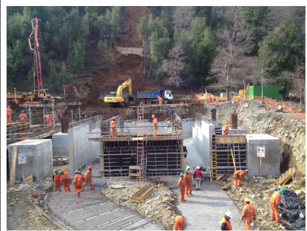
Figure 19: Construction process Sources: Pictures provided by LAP
