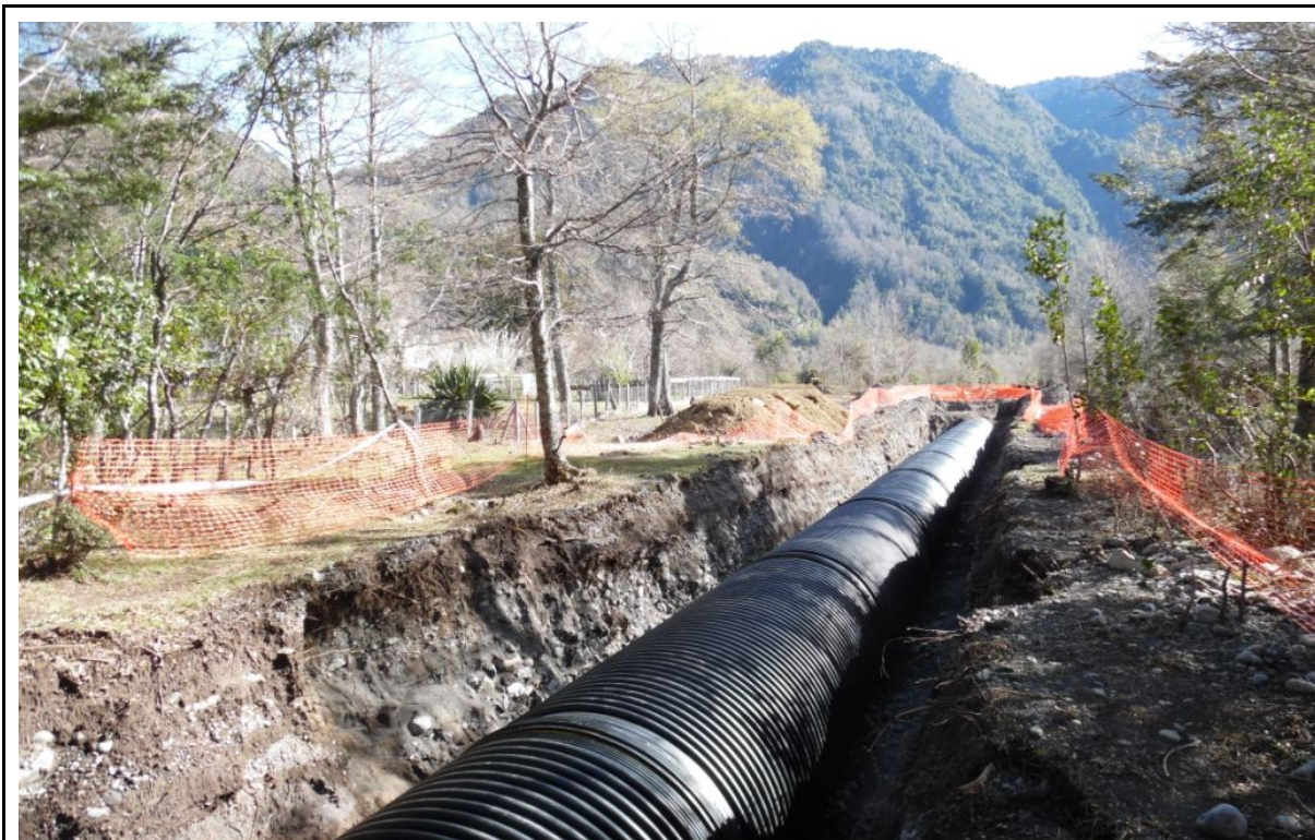
Figure 01: Pipe coming from one of the hydropower plants Sources: provided by LAP – Latin America Power
