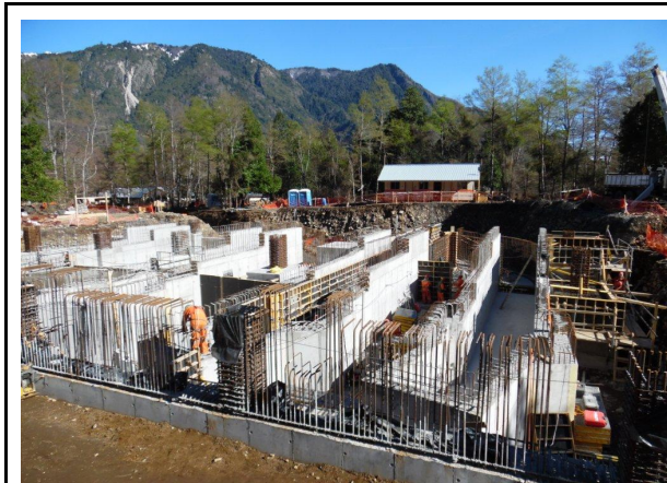
Figure 14: Construction process Sources: Pictures provided by LAP
