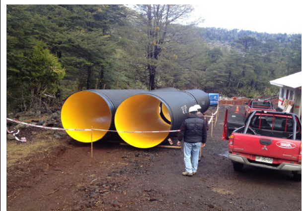
Figure 17: Construction process Sources: Pictures provided by LAP
