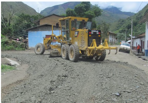
Figure 24: Rehabilitation of existing roads by project team. Source: Generación Andina S.A.C.
