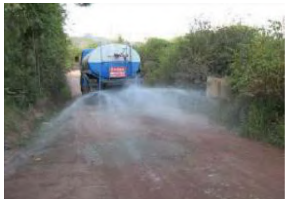
Figure 25: Units used to irrigate roads. Source: Generación Andina S.A.C.
