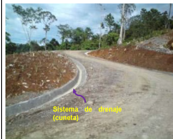
Figure 29: Drainage system built on access road. Sources: Generación Andina S.A.C.
