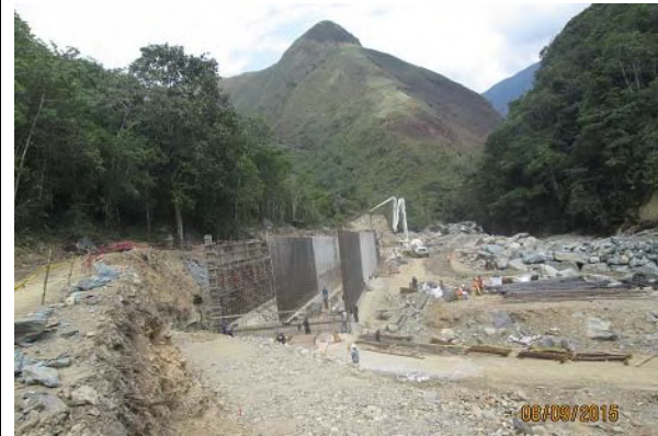
Fig 10: On-site construction. Source: Osinergmin.
