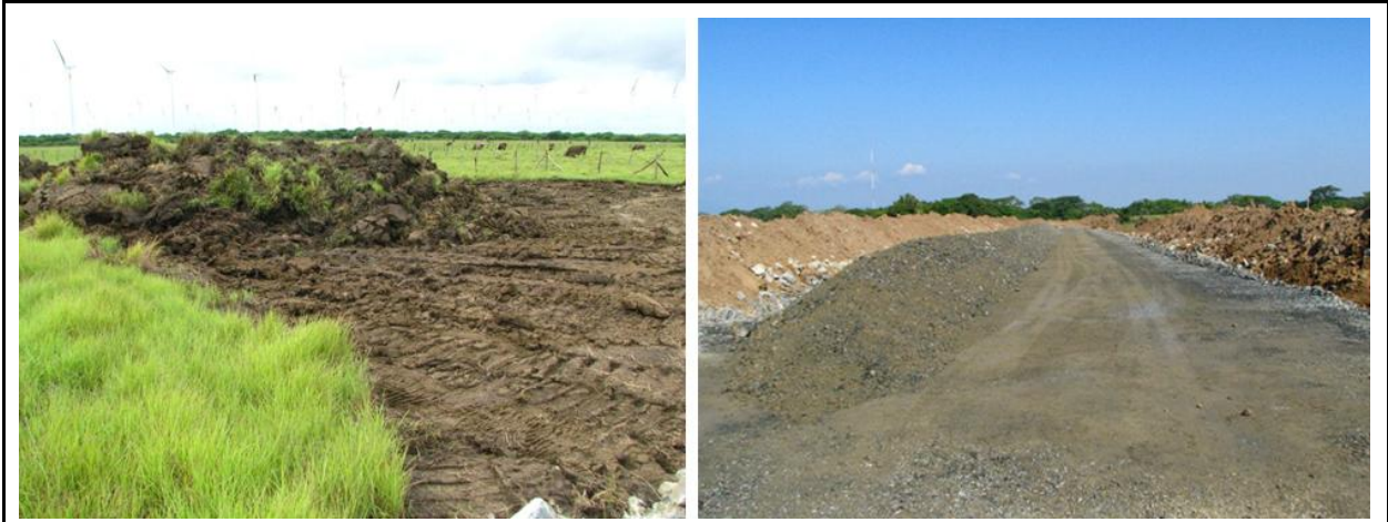
Figure 13: Reutilization of excavated soils. Sources: Anexo Fotográfico, 4-5.
