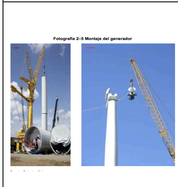
Figure 8: Construction of Turbines Sources: CSI Ingenieros, "Parque Eólico Florida Informe Ambiental Resumen (IAR)." Jul. 2012, p. 26.
