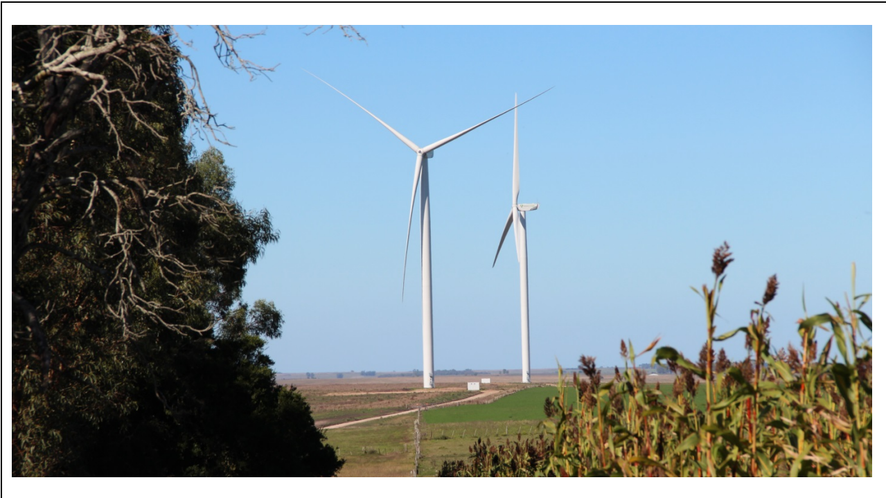
Figure 22: Wind Farm Florida Sources: Polesine S.A
