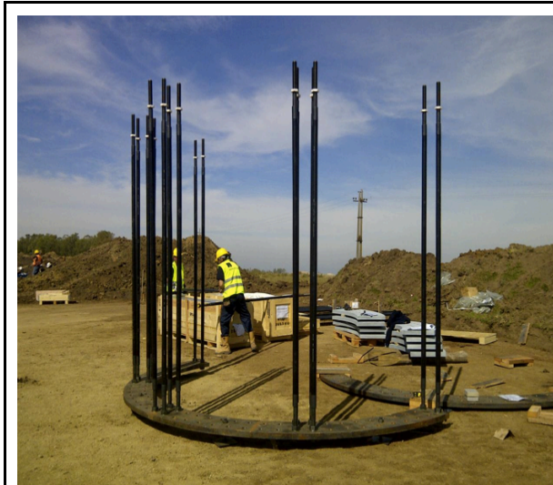
Figure 16: Florida Site where the turbines are being anchored into the ground. Sources: Piñon, A, Polesine S.A., "Componente Nacional de Inversión Parque Eólico Florida." Jul. 29 2013, p. 8.
