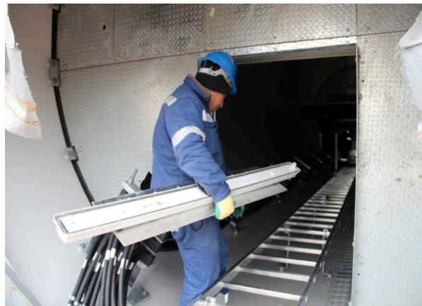
Figure 12: Trimec where assembling the turbines takes place Sources: Piñon, A, Polesine S.A., "Componente Nacional de Inversión Parque Eólico Florida." Jul. 29 2013, p. 4.
