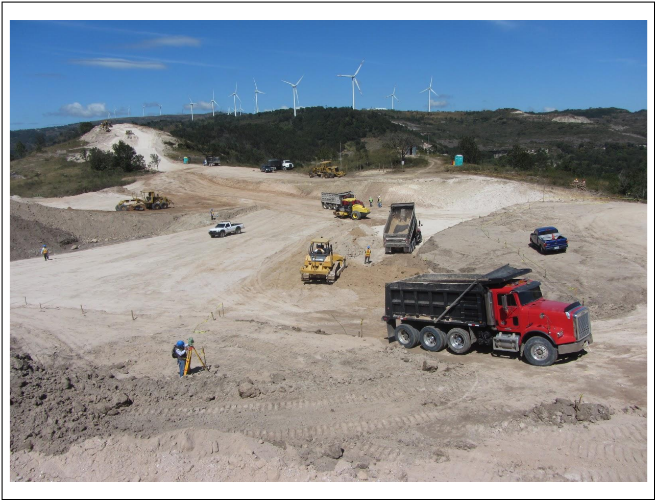
Figure 04: Construction process. Source: EEHSA.
