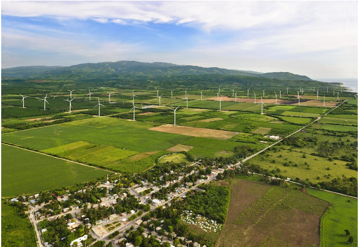
Figure 01: Wind farm and local context /Source: EGE Haina CMD project design document
