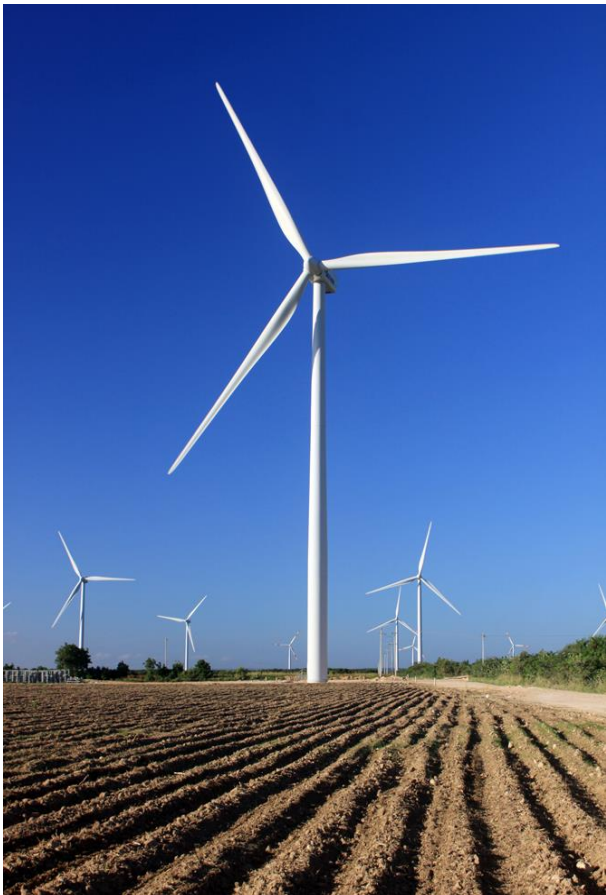
Figure Figure 40: General view of Los Cocos windfarm. / Source: EGE Haina
