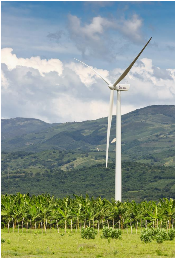
Figure Figure 41: General view of Los Cocos windfarm. / Source: EGE Haina
