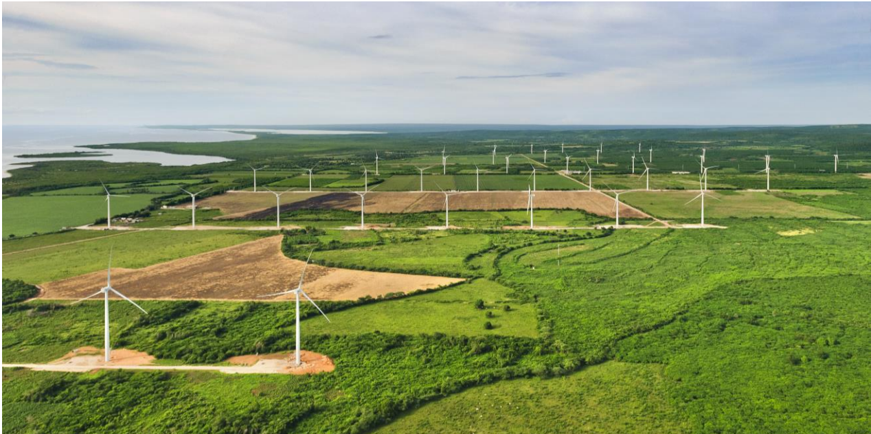
Figure 39: General view of Los Cocos windfarm. / Source: EGE Haina
