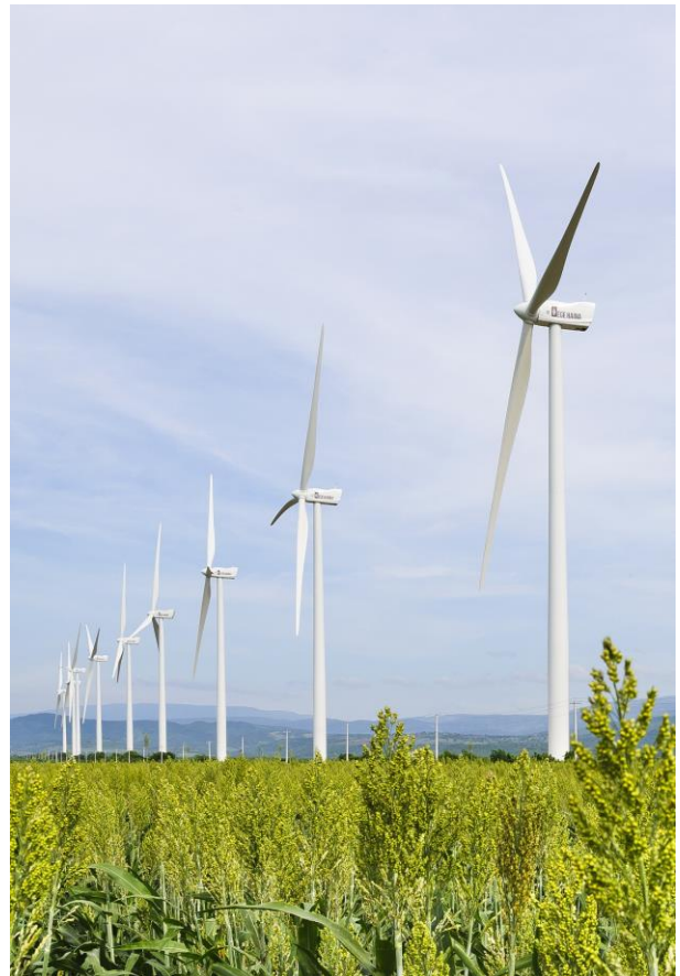
Figure 37: General view of Los Cocos windfarm. / Source: EGE Haina
