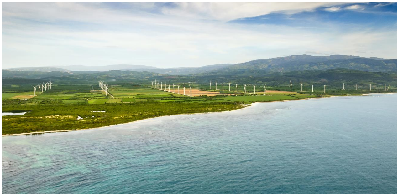
Figure 38: General view of Los Cocos windfarm. / Source: EGE Haina
