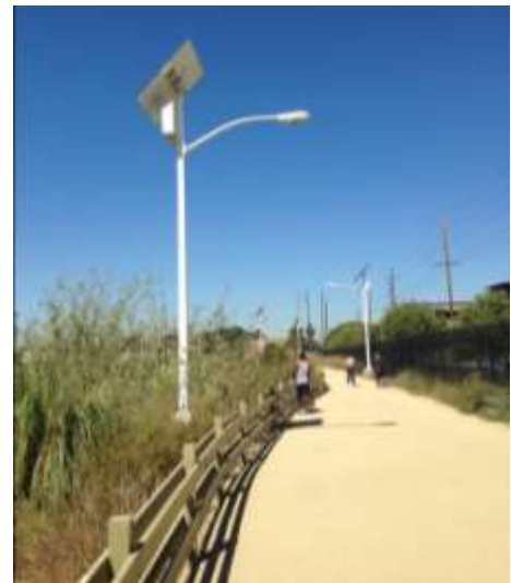
Fig.14: Security lighting zones along the pedestrian walkways were established, with a total of 41 lights equipped with solar panels (source: Prof. Pollalis)
