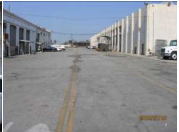
Fig.18: 100% of the site’s surface was covered with impervious material (source: material submitted for Envision rating)
