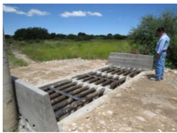
Figure 18: Depicts how infrastructure stops cattle passing from one property to another - Drainage and Passageways Enel Green Power, "Dominica I Relacionamiento con las comunidades," (presentation Jan 23 2013), México, 41.
