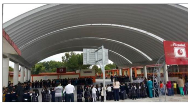
Figure 21: Children pose for a picture; the children are some of those who benefited from the new roof installations in the civic centers. Sources: Enel Green Power, "Dominica I Relacionamiento con las comunidades," (presentation Jan 23 2013), México, 40.
