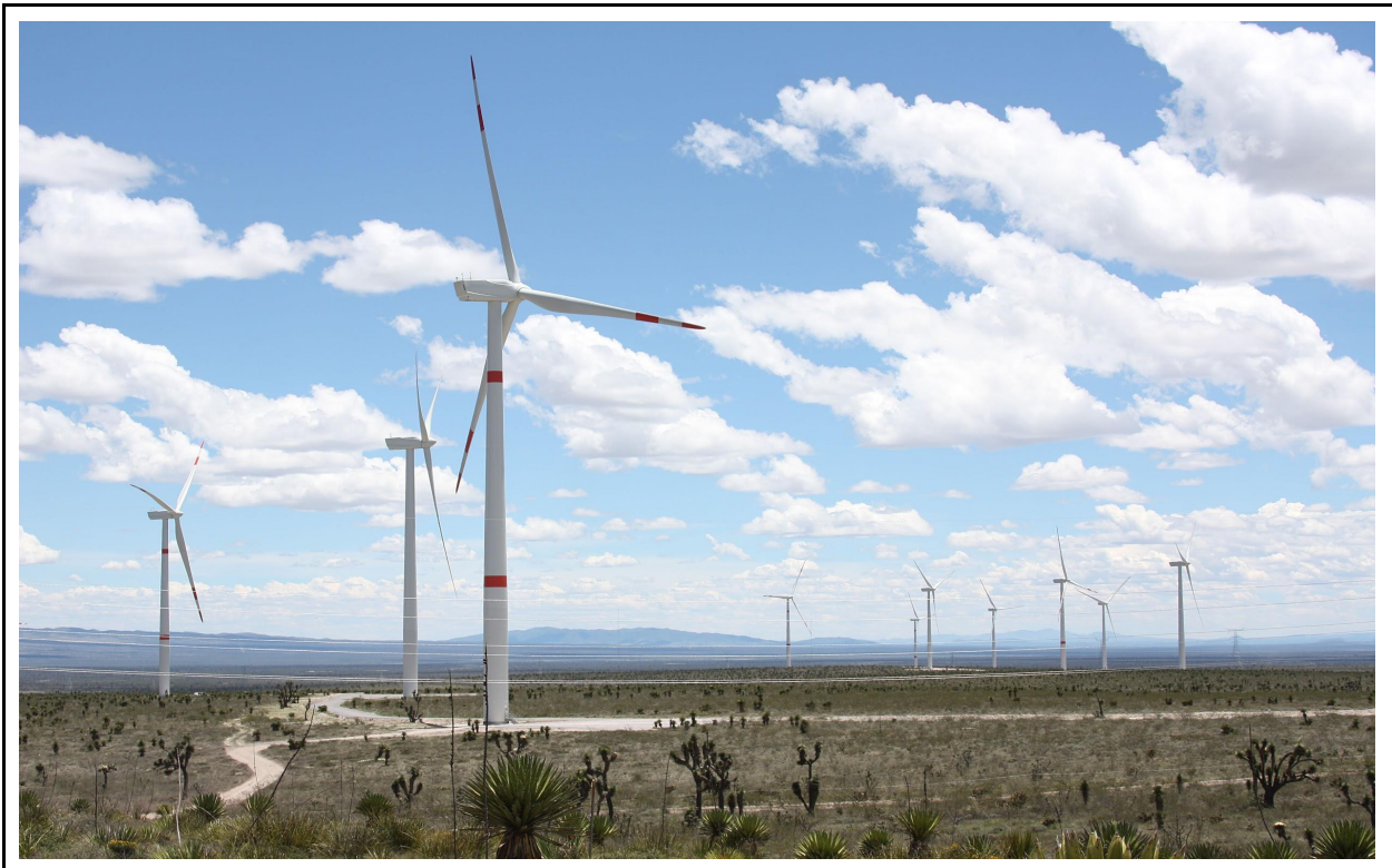
Figure 1: General view of the project Sources: Enel Green Power, "Evidencia Fotográfica [Photographic Evidence]"
