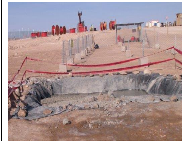
Figure 14: Permeabilized Concrete pool to prevent soil and water contamination Sources: Solarpack
