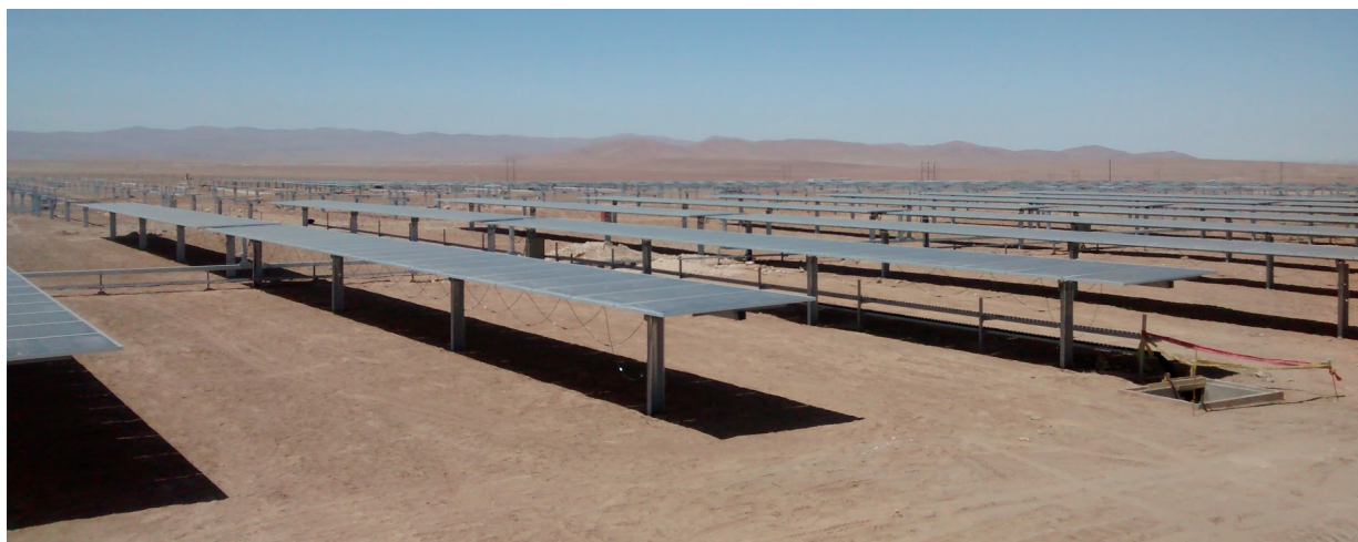
Figure 03: Overview of the plant Sources: Solarpack
