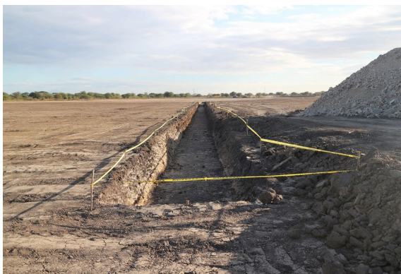
Figure 31: Excavation of Drainage System during construction phase. Sources: Anexo Fotográfico .
