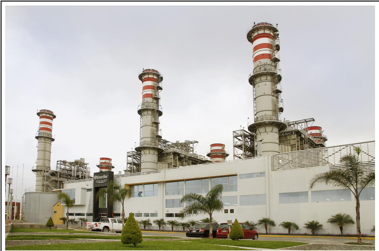
Figure 01: General view of the project. Source: EnerSur.
