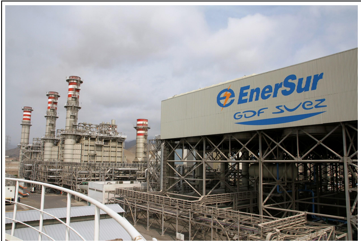
Figure 05: General view of the project. Source: EnerSur.
