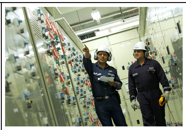
Figure 10: Work within the plant. Source: EnerSur.
