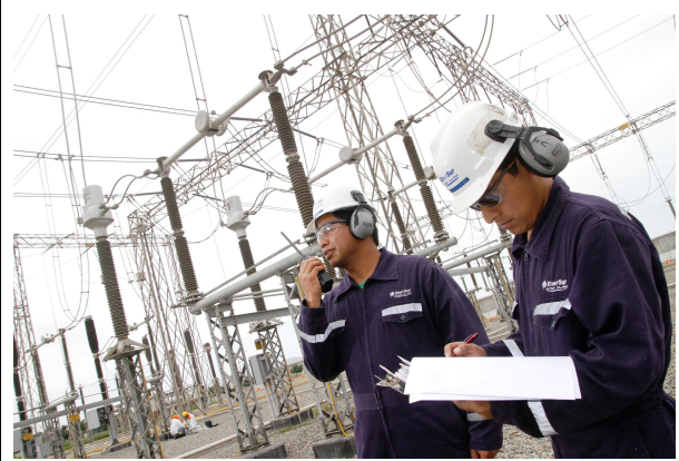
Figure 12: Work within the plant. Source: EnerSur.
