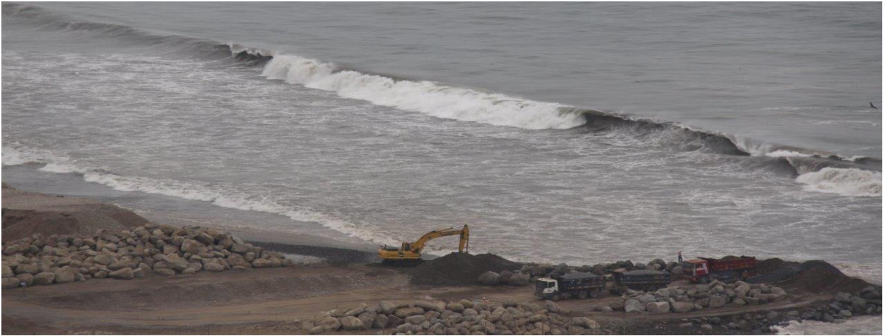
Figure 30: General view of the construction site/ Source: Proinversion
