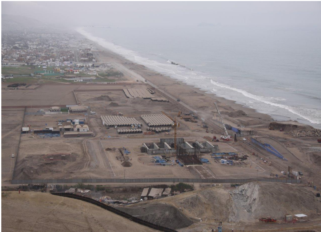
Figure 01: General view, construction process/ Source: Proinversion
