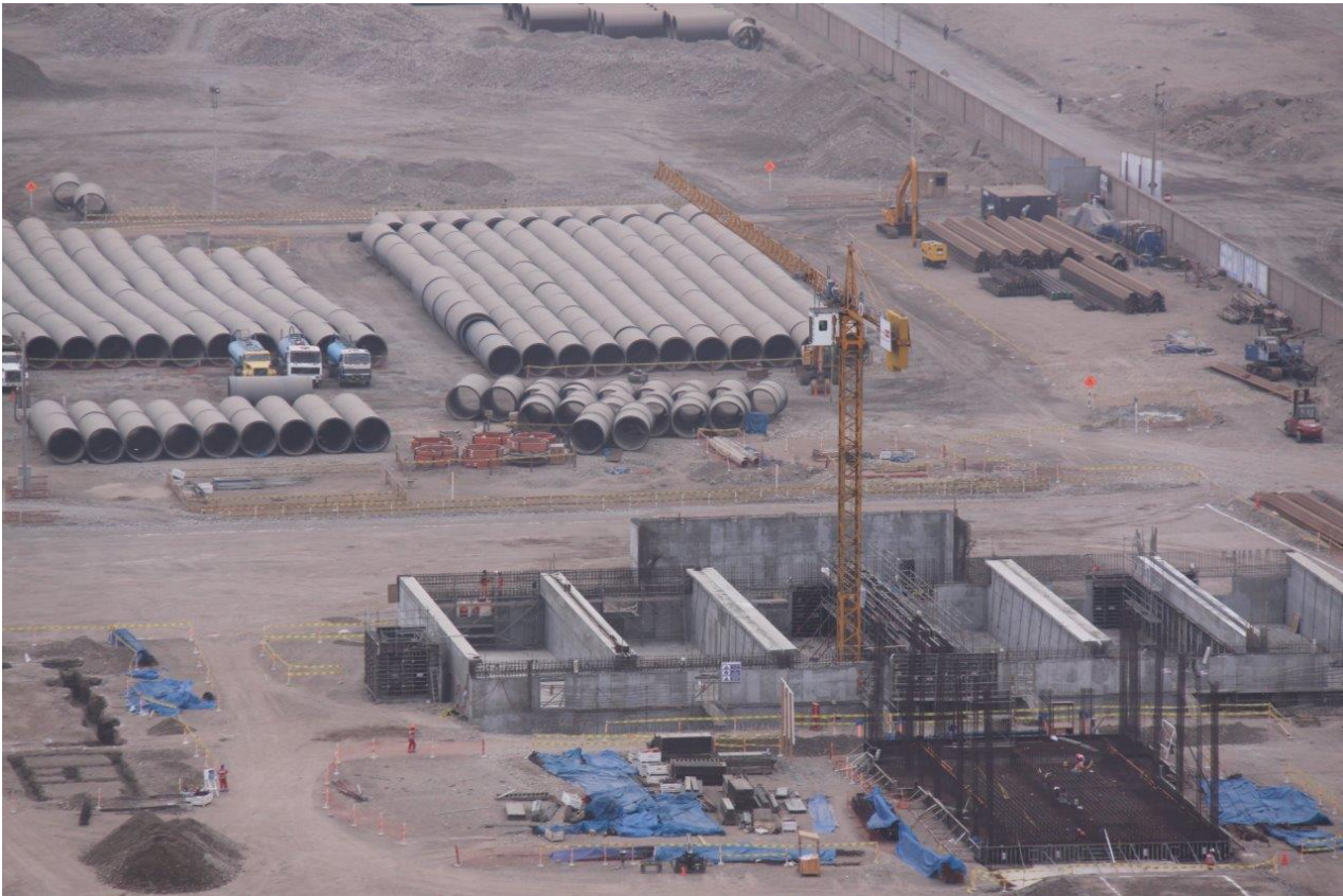
Figure 29: General view of the construction site/ Source: Proinversion
