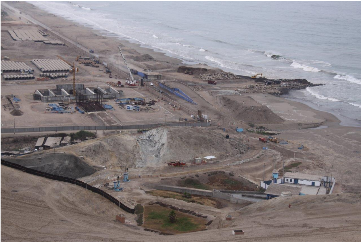
Figure 31: General view of the construction site/ Source: Proinversion
