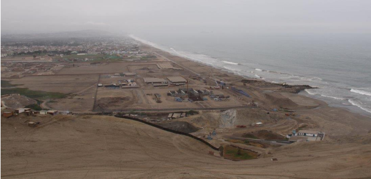
Figure 28: General view of the construction site/ Source: Proinversion
