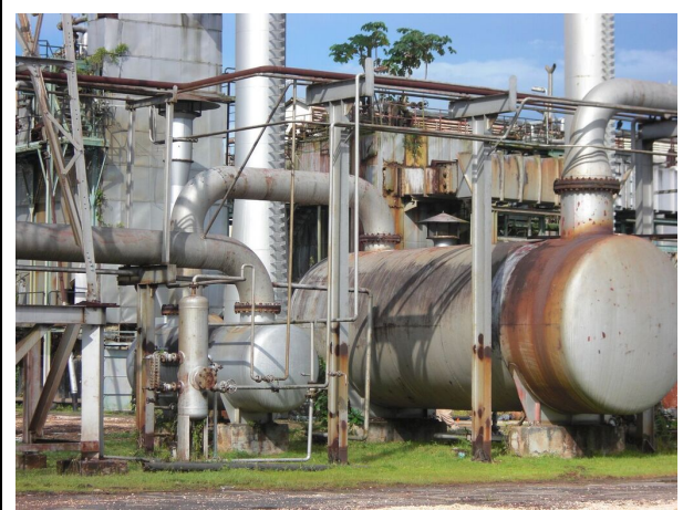
Figure 17: Fire Stack Sources: Fire Stack, by Seven Seas Water
