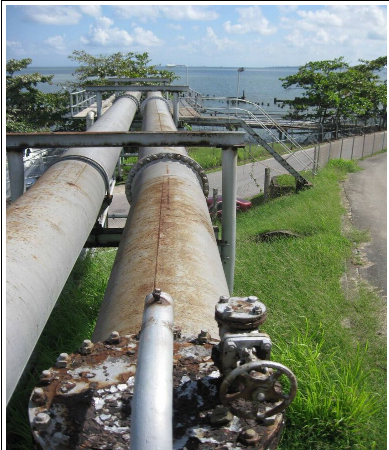
Figure 8: Pipes to the Sea Sources: Images Seven Seas Water Company
