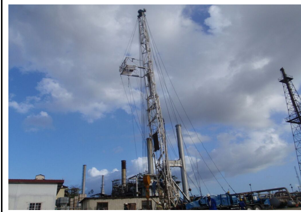
Figure 14: Oil Well Sources: Oil Well, Dropbox, delivered by Seven Seas Water
