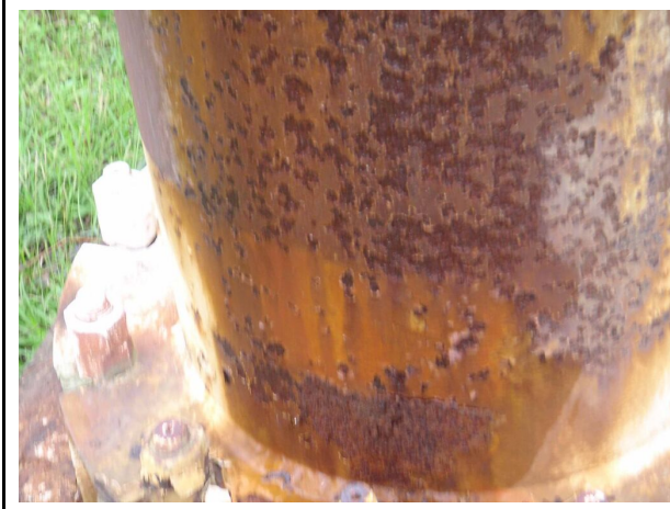
Figure 21: Structural Photos before making Plant Sources: Structural Photos, Seven Seas Water
