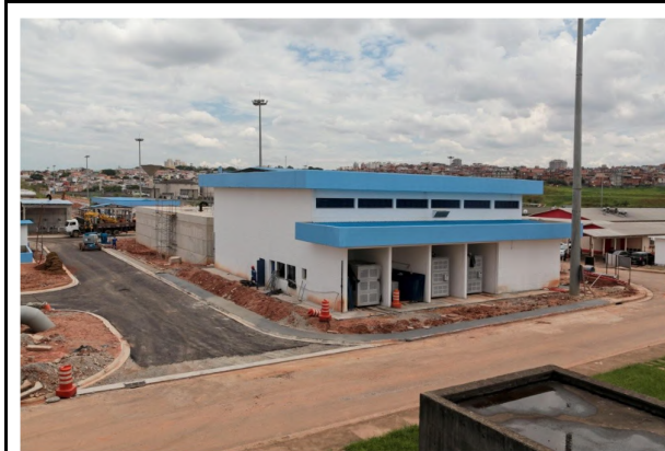
Figure 17: High pressure pump station. Sources: Aquapolo Ambiental, Apresentação geral.
