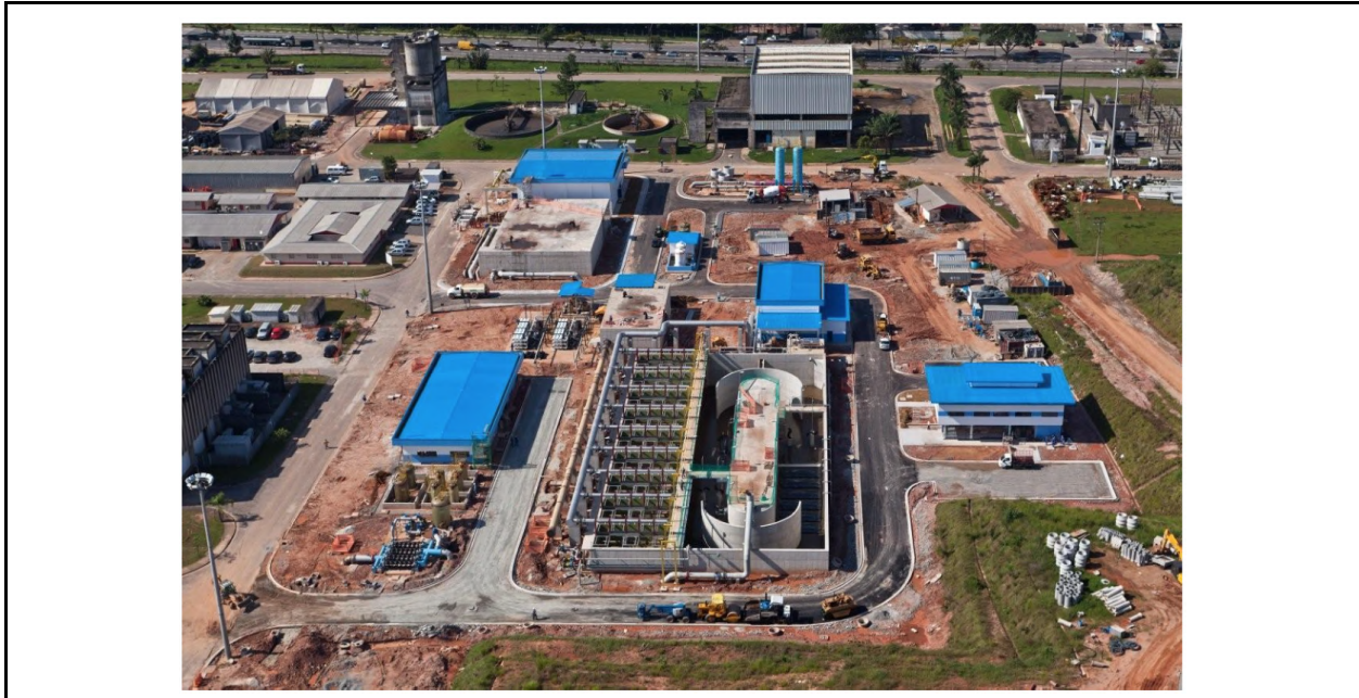
Figure 16: Construction phase, January 2012. Sources: Aquapolo Ambiental, Apresentação geral.
