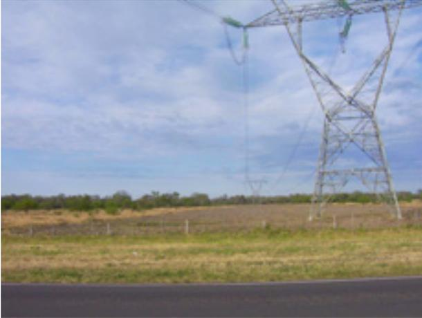
**Figure 17: Easement strip of LEAT 500kV, clear and free from trees.**
