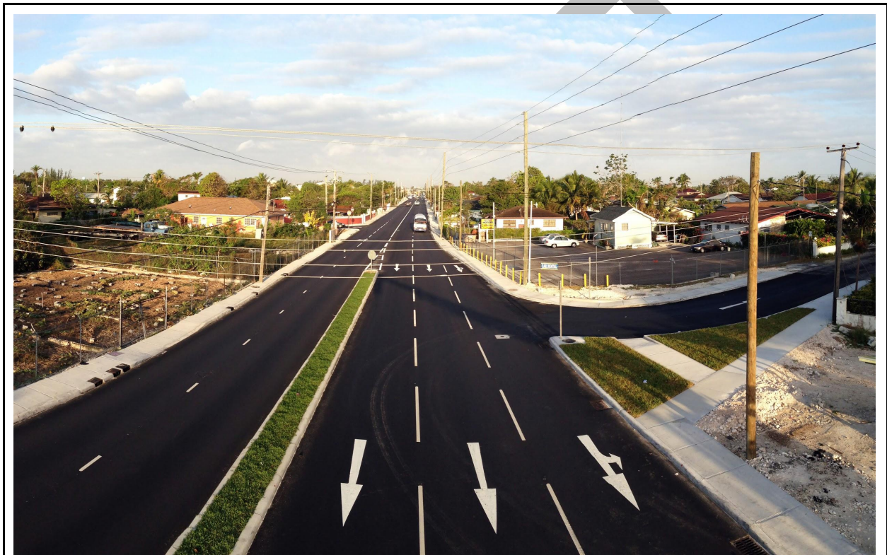
Figure 1: Completed corridor for the New Providence Transport Program Sources: Smith, Kurt, Project Execution Unit, Ministry of Works and Urban Development, October 26, 2015. Nassau, Bahamas
