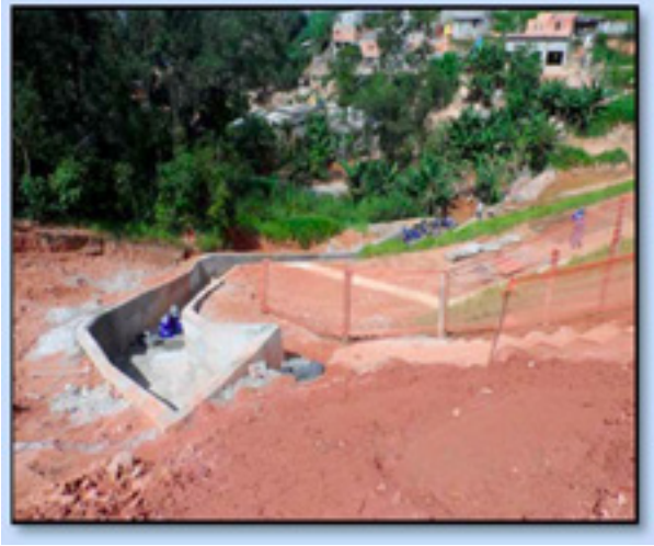
Figure 15: Permanent Drainage System
