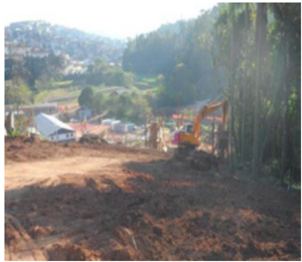
Figure 23: Supportive facilities Sources: Consórcio Cobrape Appe. Sumário Executivo. São Paulo. 2013. 68
