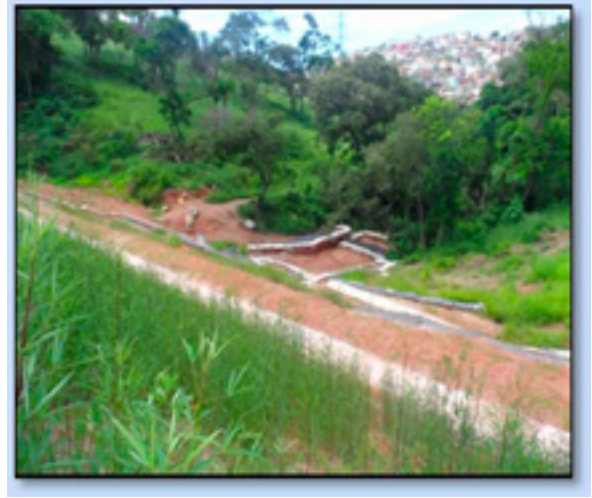
Figure 16: Provisory Drainage System
