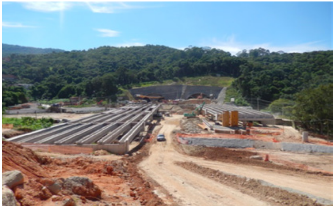
Figure 10: Construction works Sources: Consórcio Cobrape Appe. Executive Summary. São Paulo. 2015. 72
