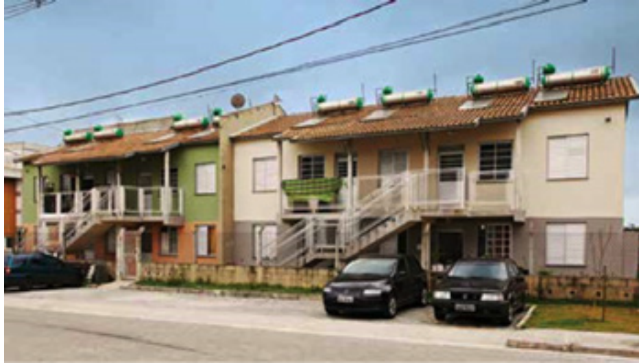
Figure 15: Solar water heaters. New housing reduced energy consumption and costs by providing houses with solar powered water heating.
