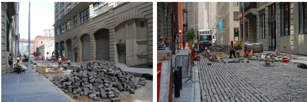
Fig.8, 9: Construction works on Washington St during Phase I
