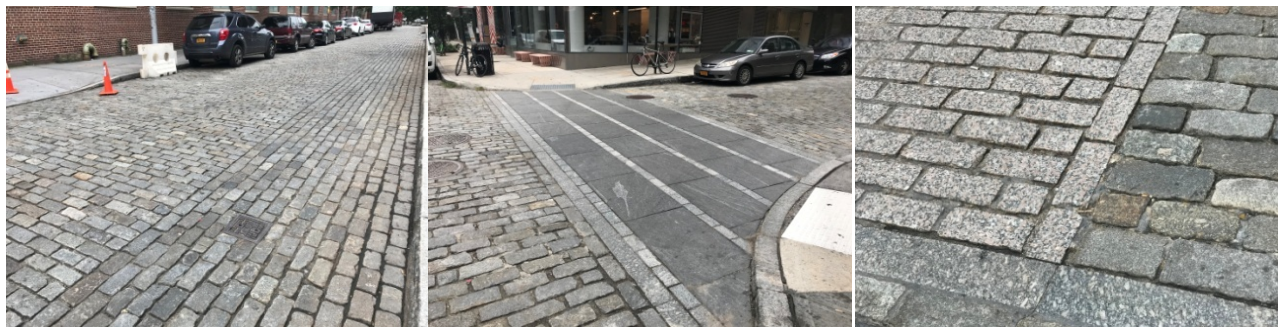
Fig. 10, 11, 12: Completed Phase I works on Water St.
