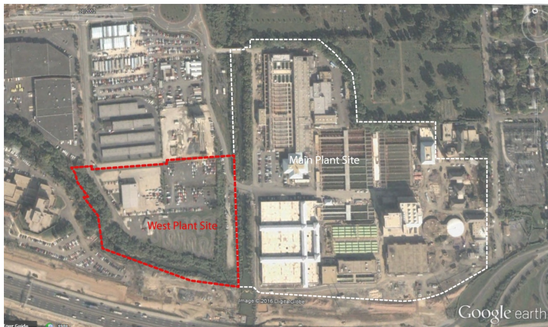
Fig. 1: AlexRenew main plant site and west site before construction
