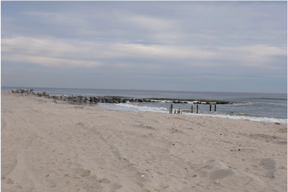
Exposed bulkhead on western area of Fort Tilden. Source: J. Rodriguez
