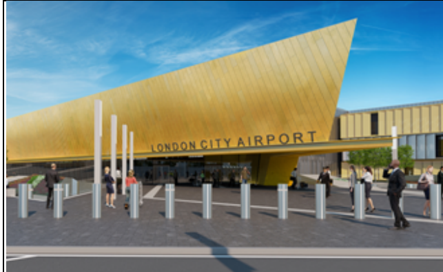
Fig. 20: Terminal front entrance (source: Bechtel)
