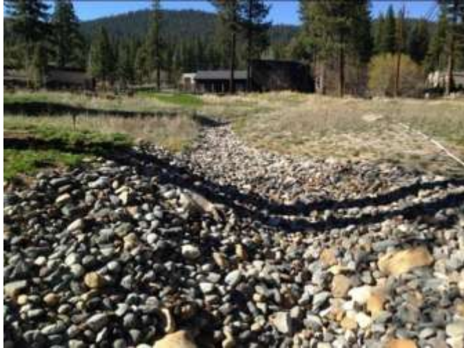
Fig.13: The water channel
