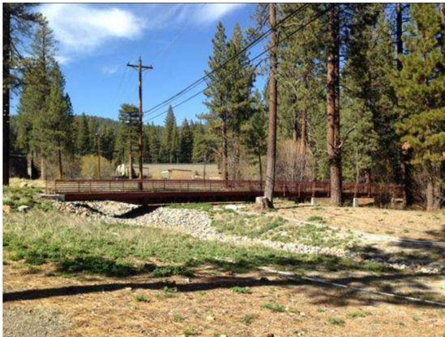
Fig.12: The new bridge made of a recycled railroad flat car
