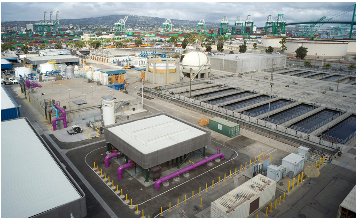
Figure 1: Terminal Island Wastewater Reclamation Plant/Photograph provided by The Walsh Group, 2017
