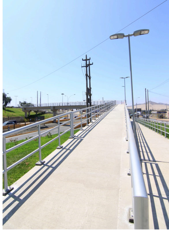
Figure 28 : View of Pedestrian Bridge Sources: Vias Nuevas de Lima
