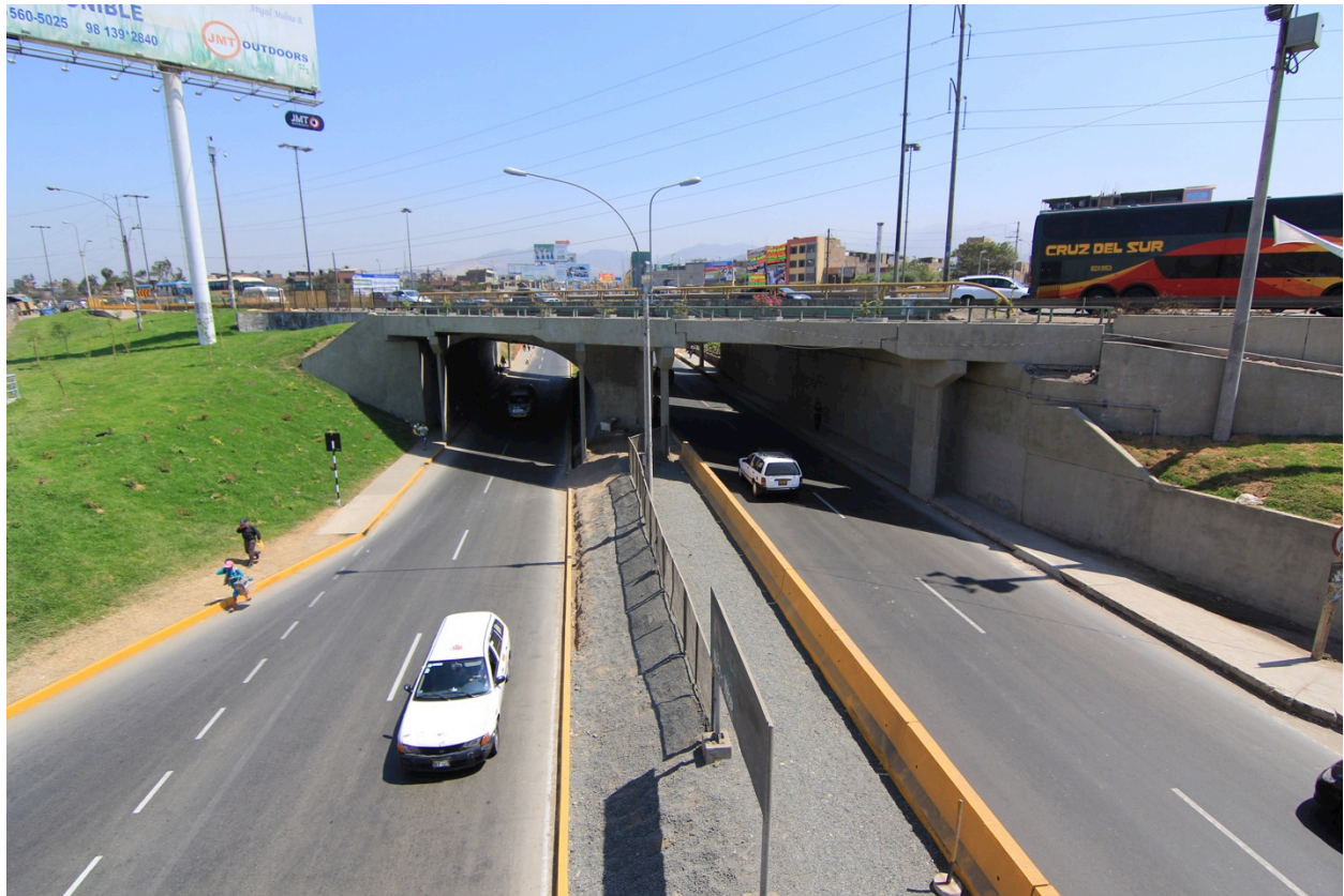
Figure 31: View of highway underpass Sources: Vias Nuevas de Lima
