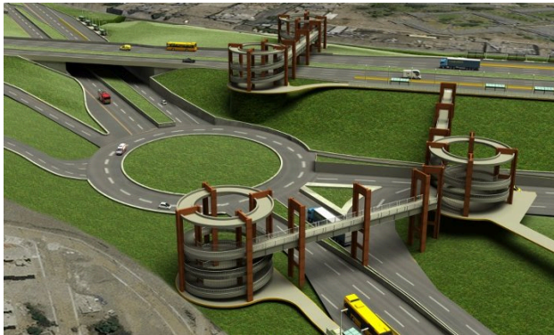
Figure 24: View of Pedestrian Bridge Sources: Vías Nuevas de Lima
