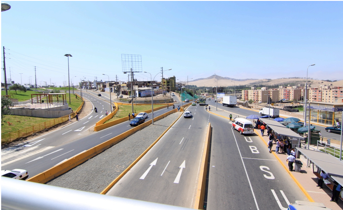
Figure 30 : View from Pedestrian Bridge Sources: Vias Nuevas de Lima
