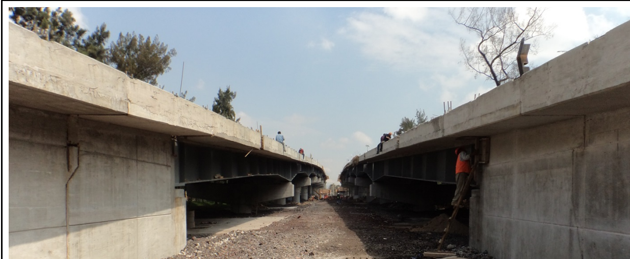
Figure 16: Revolución – Molinos Construction Site
