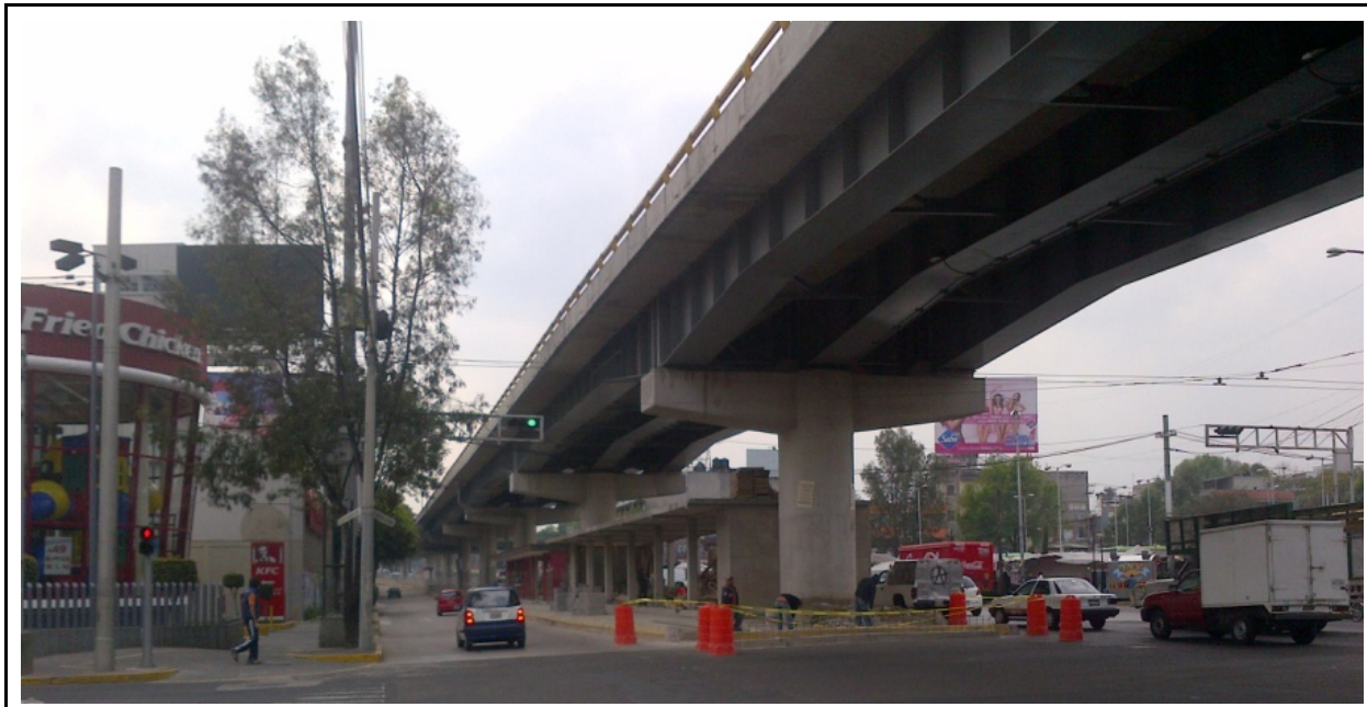
Figure 03: Image towards southern part of Revolution Avenue. Sources: Photographic Report from Traffic Impact Study. P.1
