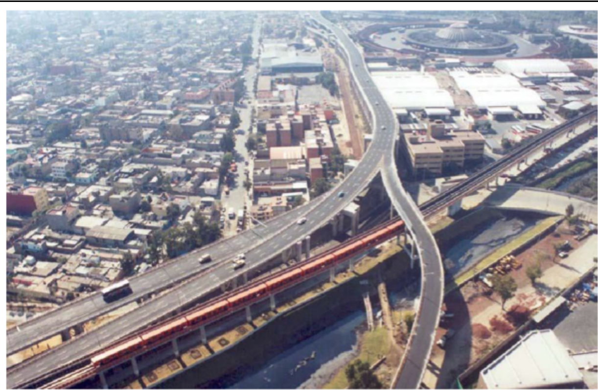
Figure 02: Urban bridges of Mexico City, 2005.
