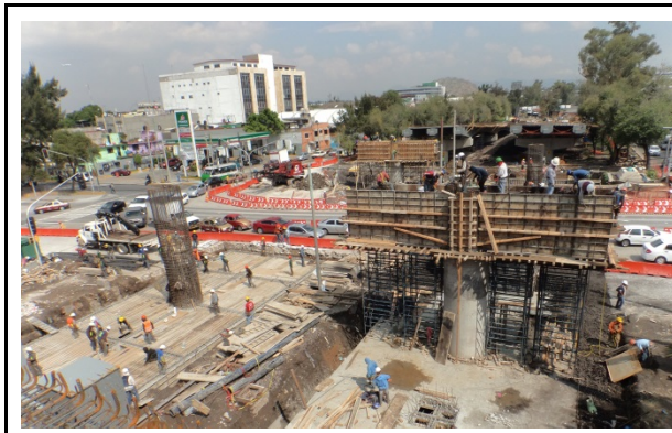
Figure 04: Bridge under construction. Sources: Photographic Report from Grupo Indi.
