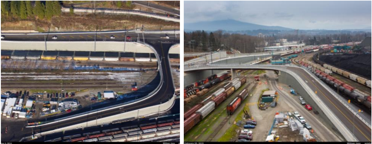
Fig. 8. Aerial views of the overpass at the Neptune/Cargill terminal entrance (Source: PMV)
