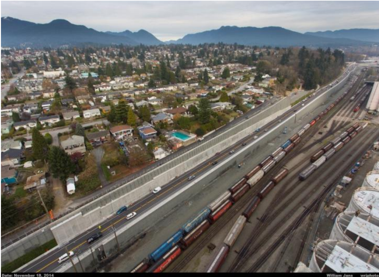
Fig. 4. Aerial view of the project (Source: PMV)
