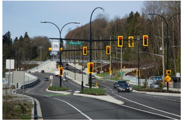
Fig. 12. LLR at-grade crossing with E 3rd Street looking west (Stantec)
