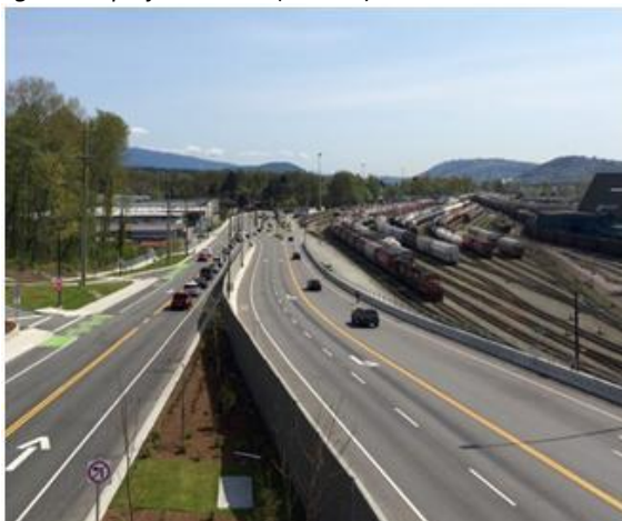
Fig. 6. Driving on the east part of LLR (Stantec)
