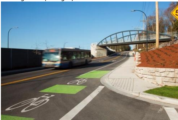
Fig. 13. Pedestrian overpass at E 3rd Street (Stantec)
